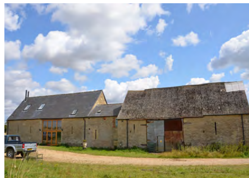
Existing Grade II Listed barns at Himley Farm
