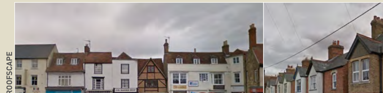
Varied and articulated roofscapes to the historic core. Projecting gables provide a sense of rhythm to the roofscape punctuated with chimneys.
