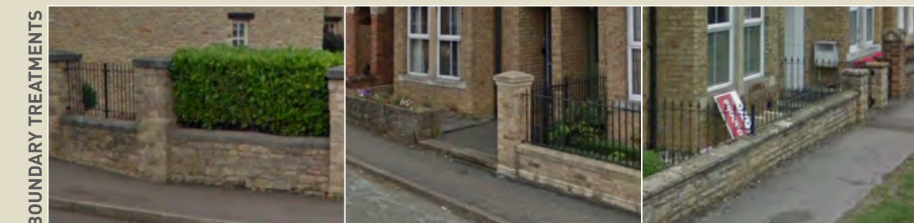
Predominantly low level walls, some with additional hedgerow or railings.
