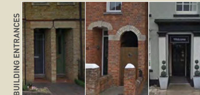
Stone headers with no canopy. Typical Georgian header and pillars.
