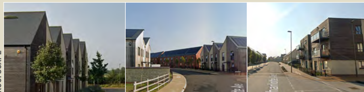
Strong rhythm and uniformity to the roofscape is common within the development to form signature frontages. Roofs are orientated (wherever feasible) to maximise efficiency for PV solar panels. Generally simple pitched roofs with no evidence of dormers or chimneys. Flat roofs to apartment buildings.
