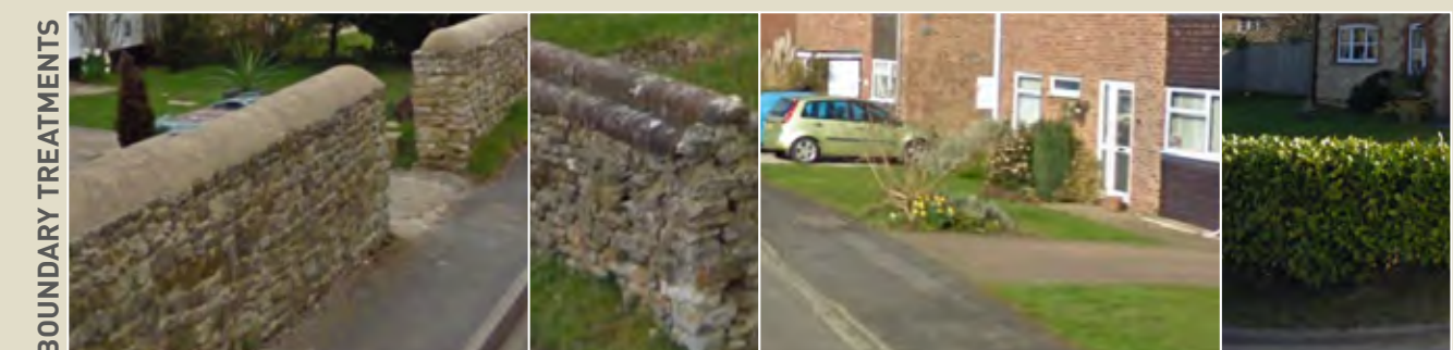
BOUNDARY TREATMENTS Predominantly low walls to the older part of Ardley Predominantly open with shrub planting and some use of hedgerows in the newer areas of Ardley
