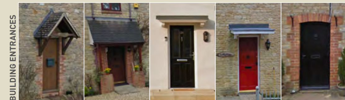
BUILDING ENTRANCES Pitched door canopies Flat door canopies Arched brick header and quoins to door with no canopy
