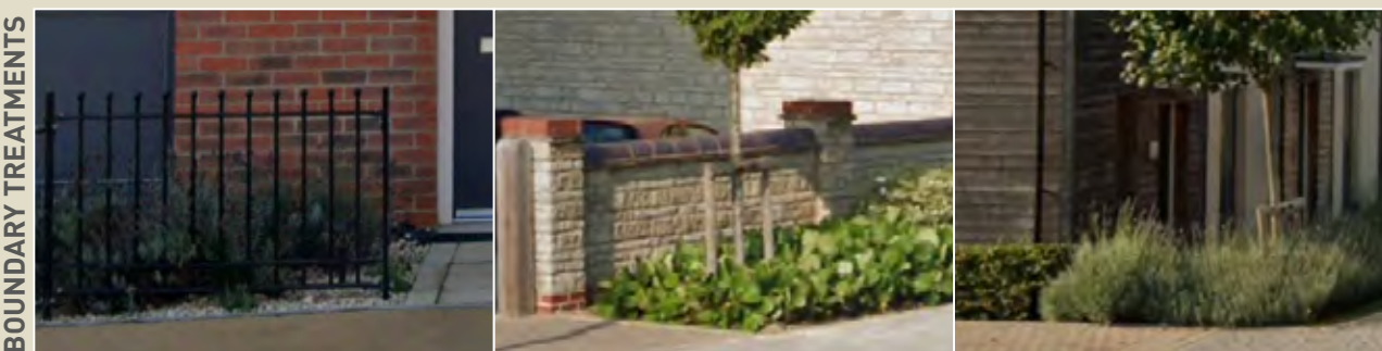
Railings and shrub planting to primary street. Low stone walls and shrub planting to parking court entrances. Low level shrub and hedge planting with some trees within the front gardens.
