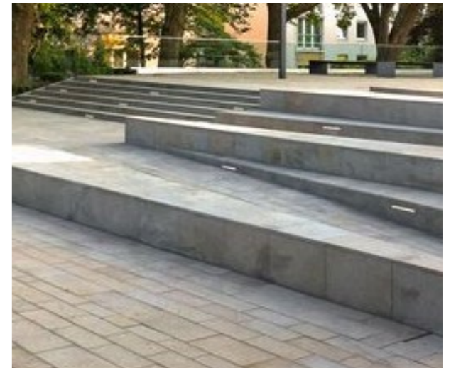
STEPPED AND ACCESSIBLE RAMP ACCESS
