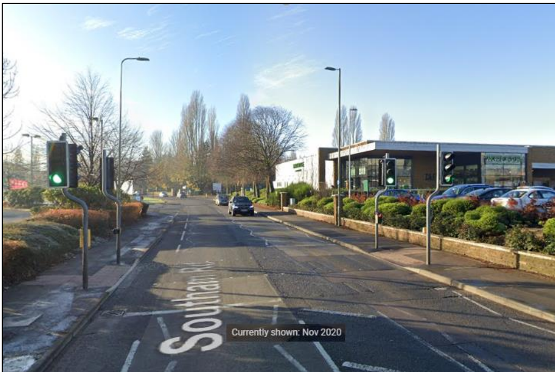
Image 2: Signalised Toucan Crossing 120m North of the Site Access
