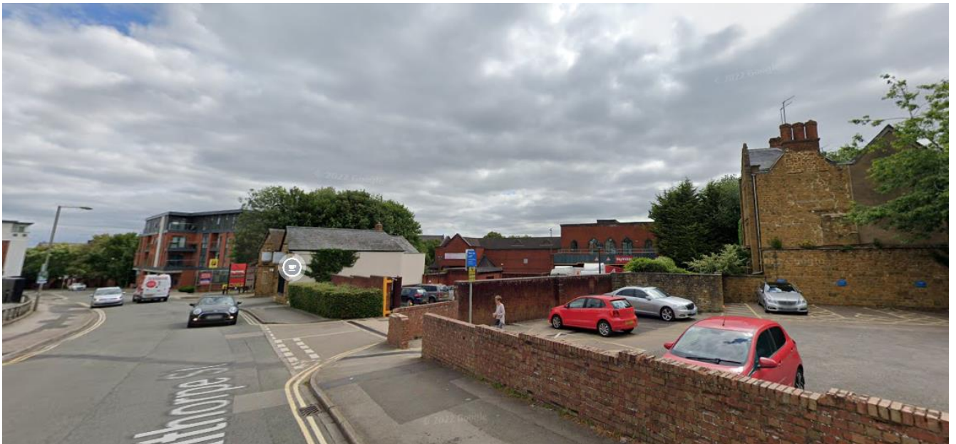
View looking north along Calthorpe Street with the Grade II* Calthorpe Manor on far right and its locally-listed former gate lodges centre left. If the proposed development is approved and built, almost the whole of this view will be dominated by 4- and 5-storey blocks of flats, resulting in significant harm to the setting of these important historic buildings
