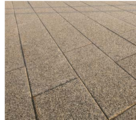
PAVING TYPE 3 Marshalls Modal Priora Mid-grey Granite, Mixed Sizes
