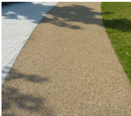
PAVING TYPE 4 Aggagrip Terraco Resin Bound Gravel, Dorset Gold, 6mm Gravel
