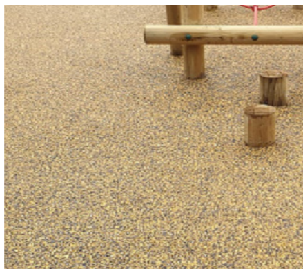
PAVING TYPE 9 DCM Wetpour Play Surface 1-3mm Colour Varies
