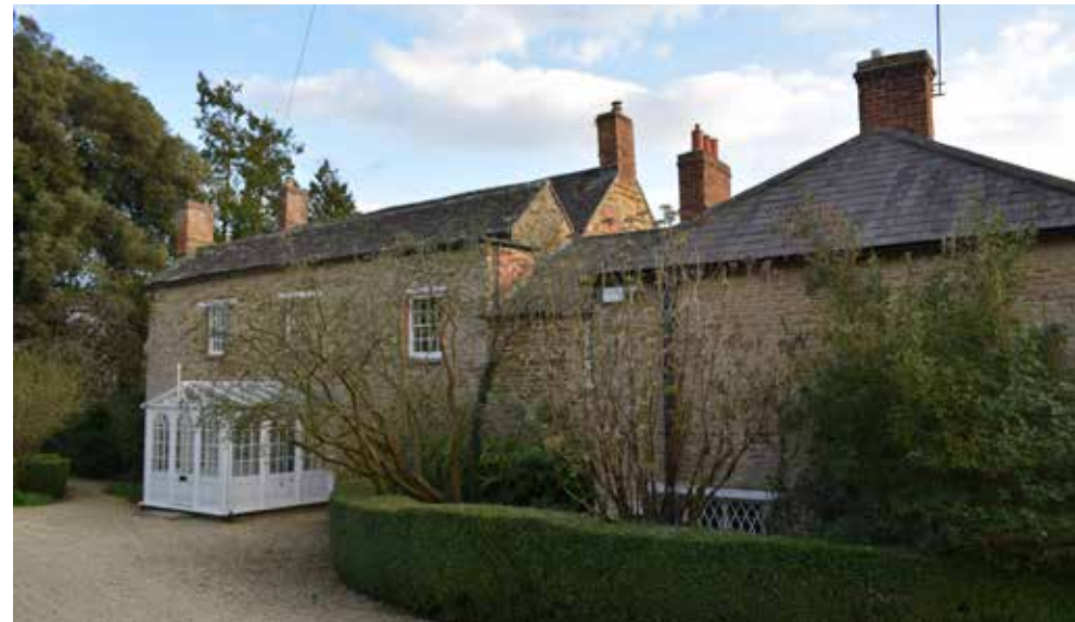
Fig 18: North elevation from the northwest showing the main range with modern timber porch the two-storey extension and the former service wing
