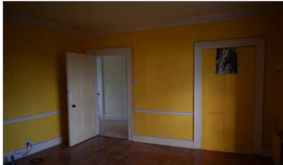
Fig 34: Eastern wall of the bedroom with the entrance door and a door to a narrow cupboard simple skirting, dado and cornice
