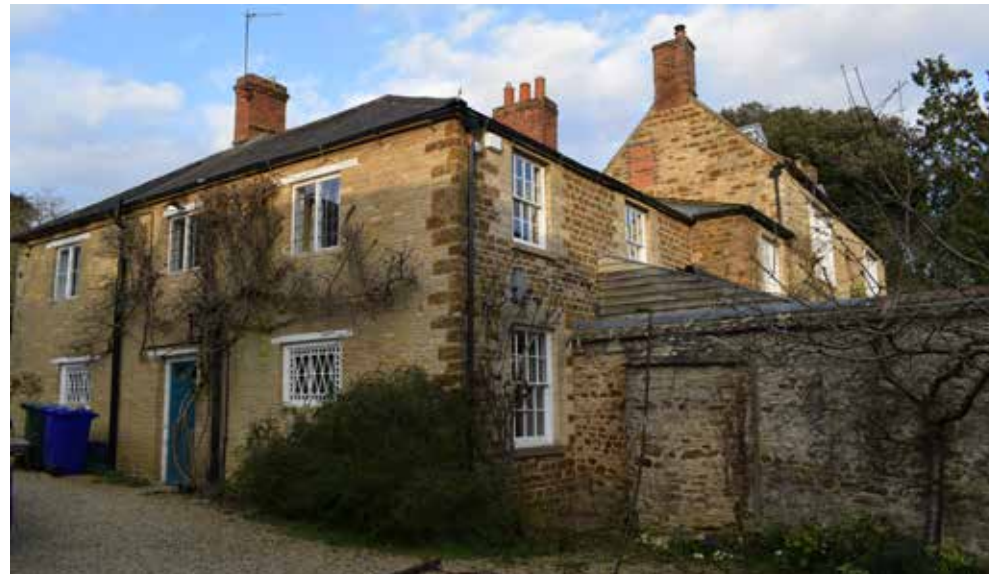
Fig 21: View of the former service wing from the south west showing the symmetrical west elevation of the north south range with the wrought iron casement windows, and the rear (south) elevation with sash windows and the lean-to extension, and the roof of the conservatory over the wall running south west from the elevation.
