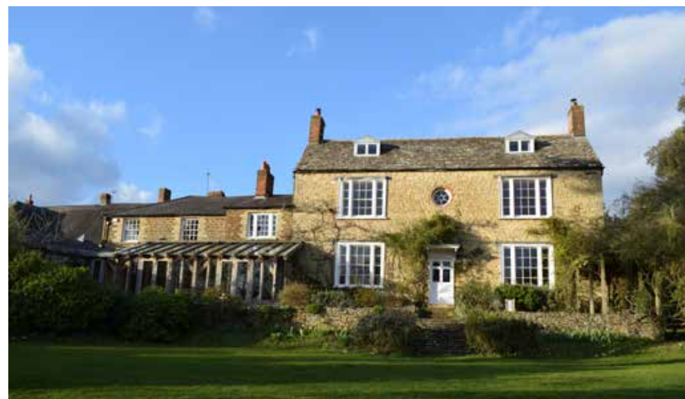
Fig 19: Rear (south) elevation of the house with symmetrical elevation and former service wing to the west with new conservatory and reintroduced dormers to the roof.
