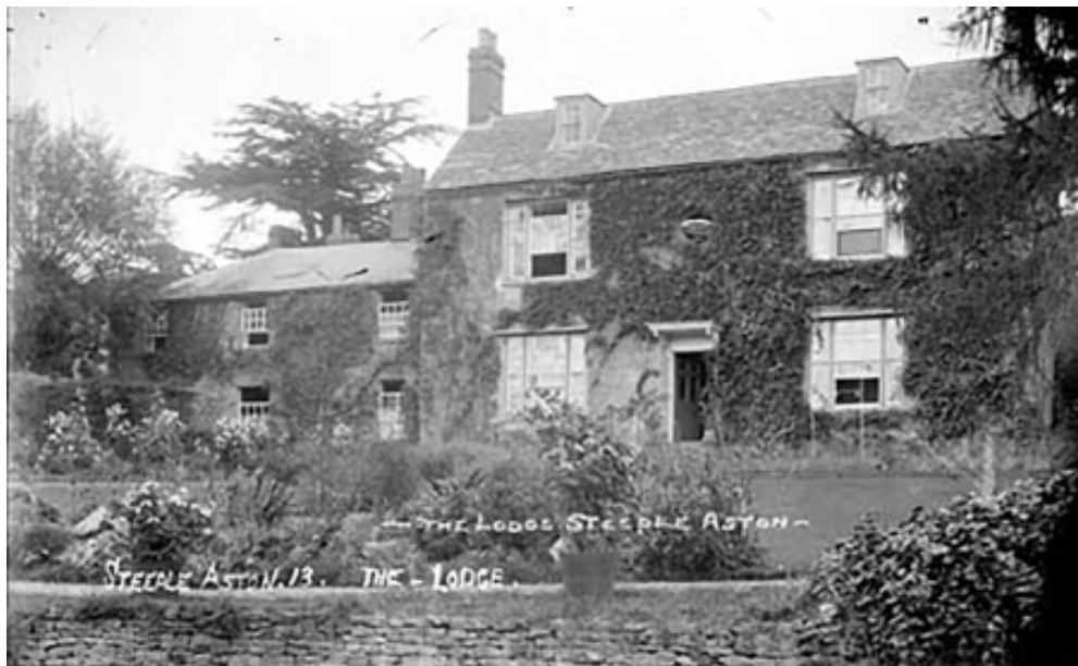
Fig 12: Packer Collection, Oxford History Centre. Photographed c. 1900 – Note tall dormers to the south roof slope and no bay to the ground floor of the service (west) wing with extension above. Elevation appears rendered – list description refers to stucco
