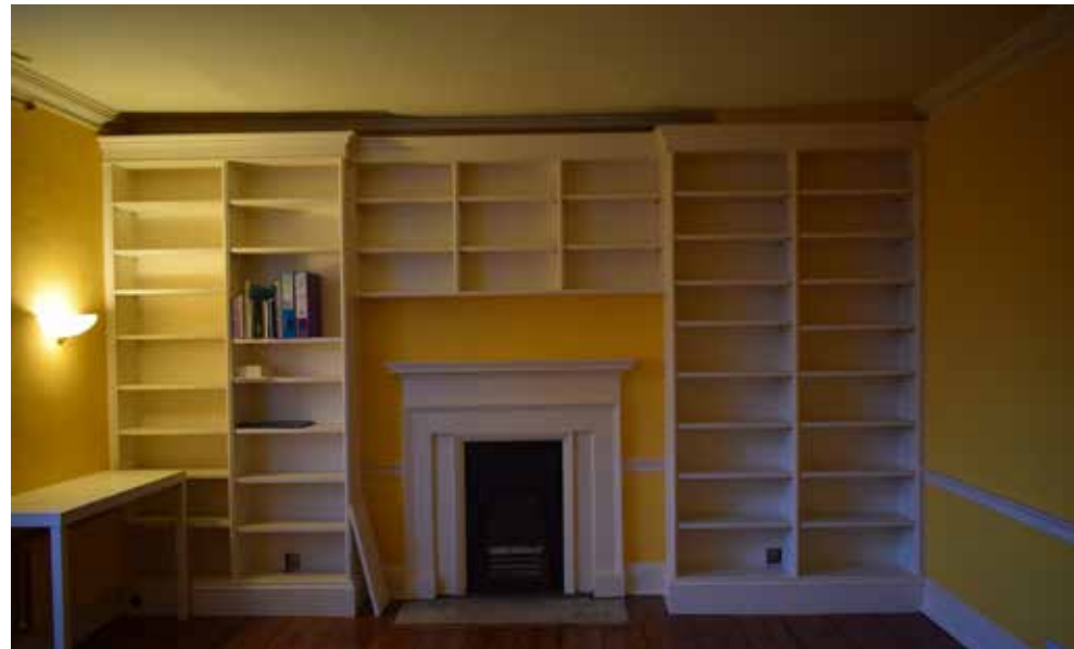
Fig 35: Western wall showing the simple skirting, dado and cornice, and the centrally placed fire surround and bookshelves which are proposed to be removed. The opening is proposed to the right-hand side of the fireplace surround
