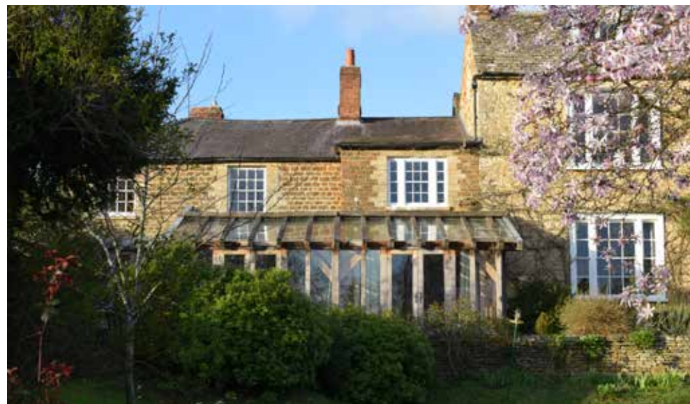
Fig 22: View of the rear (south) elevation of the former service wing showing the 8 over 8 sash windows to the first floor
