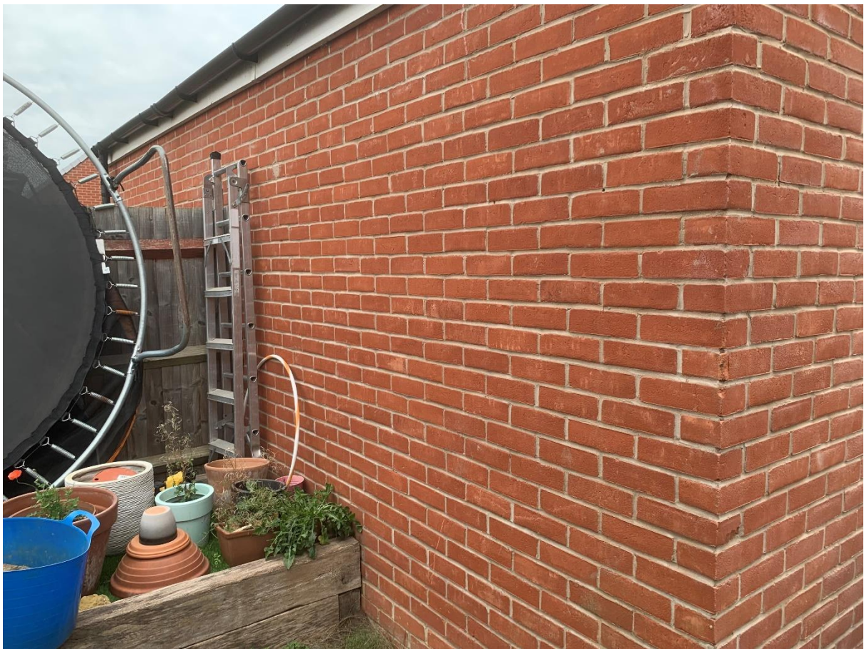
Image 16: Wall where window will be installed
