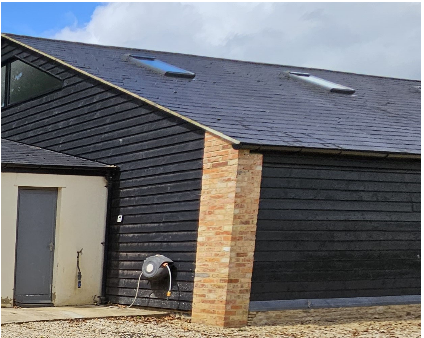
Photo 1 – Existing Outbuilding – Timber Clad walls and Fibre slate tiled roof.
