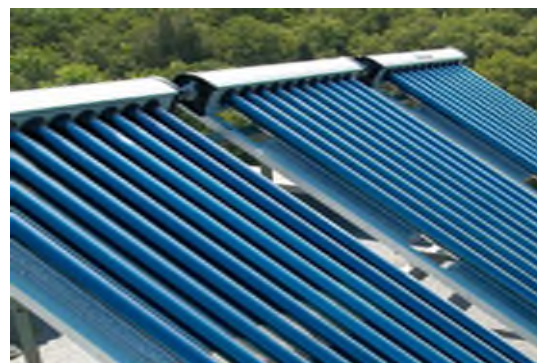
Figure 10: Solar thermal hot water panels.
