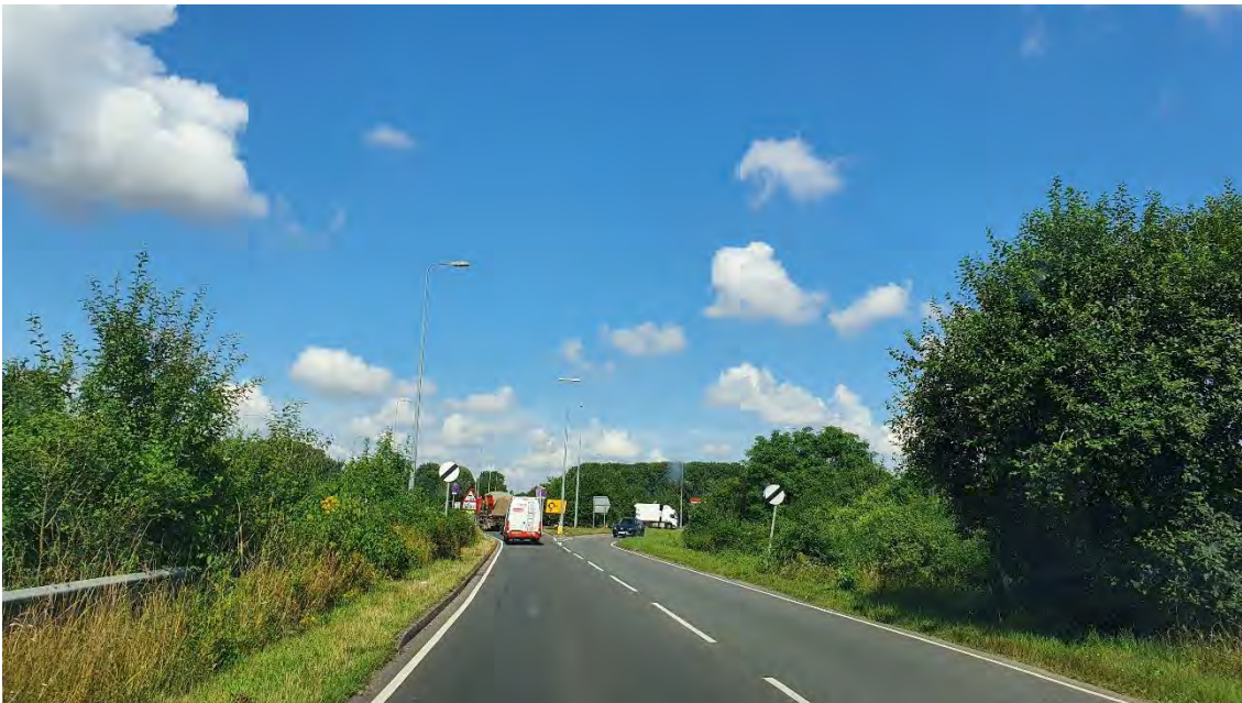
Figure 1: Existing lighting on northbound B4100 approach to Baynards Green roundabout.
