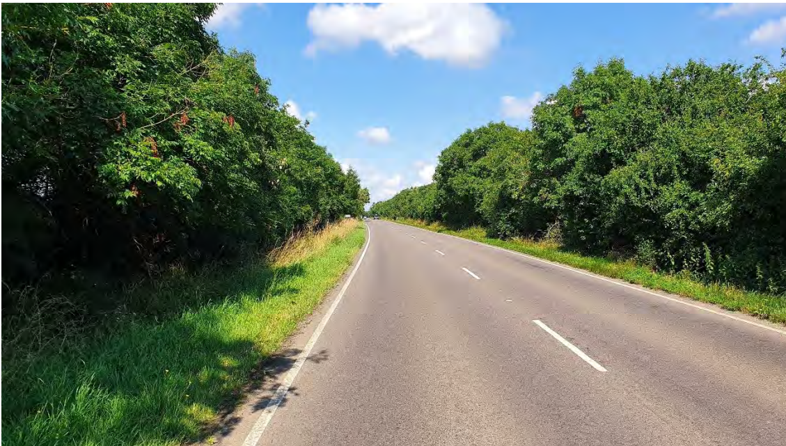
Figure 1: Existing B4100 on northbound approach to proposed roundabout.
