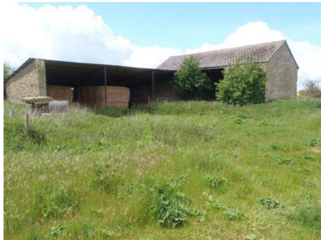
Barns in western part of site
