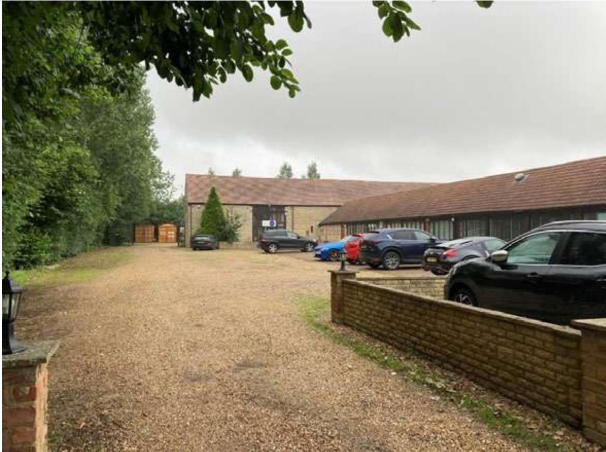
Plate 1: Entrance to the converted Barn at the former Baynard's Green Farm
