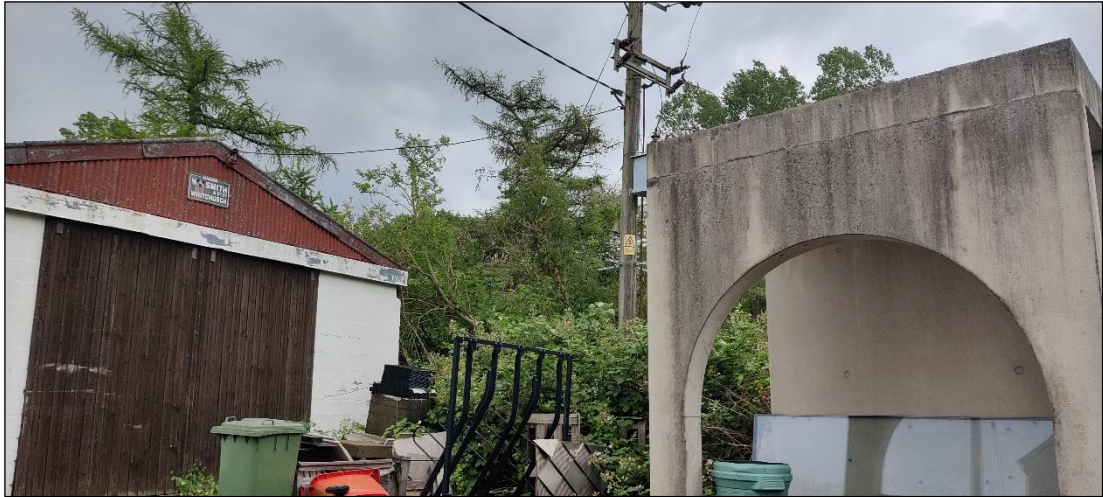
Photo 4 View of outbuildings associated with Frieze Farmhouse view north-east
