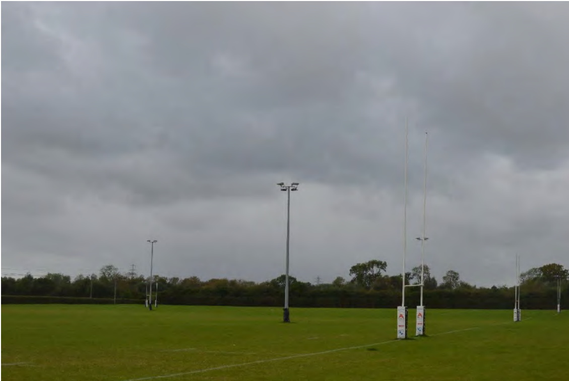
Figure 5.4: Sports lighting luminaires used at Stratfield Brake Sports Ground. Four head arrangement.
