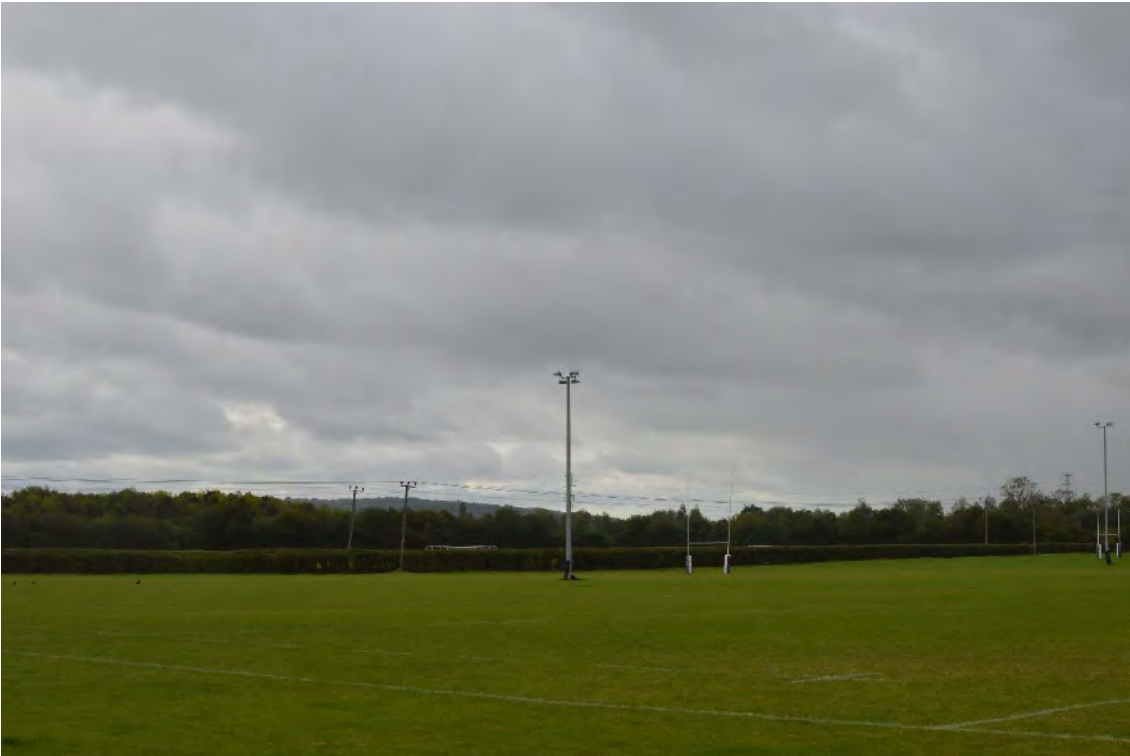
Figure 5.3: Sports lighting luminaires used at Stratfield Brake Sports Ground. Four head arrangement.
