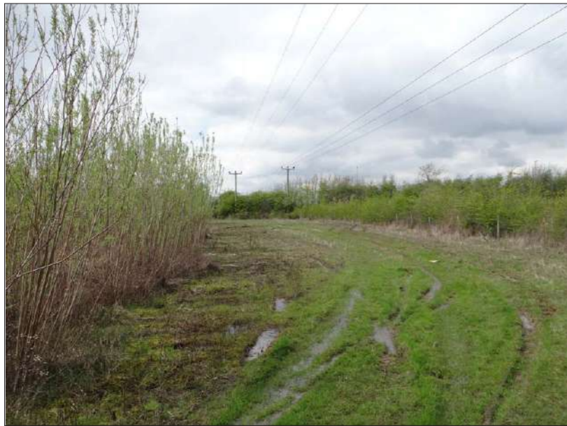
PHOTOGRAPH S2 - VIEW FROM THE NORTH EASTERN PART OF THE SITE, LOOKING WEST ALONG THE LINE OF THE OVERHEAD CABLES.
