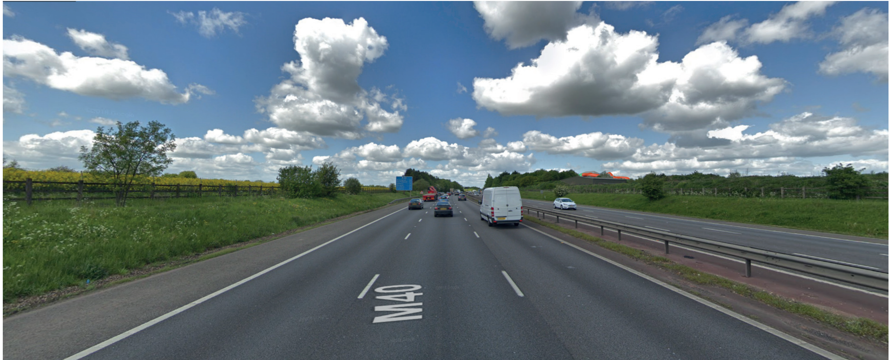
This view provides an illustration of which parts of the scheme would be seen before establishment of mitigation planting
