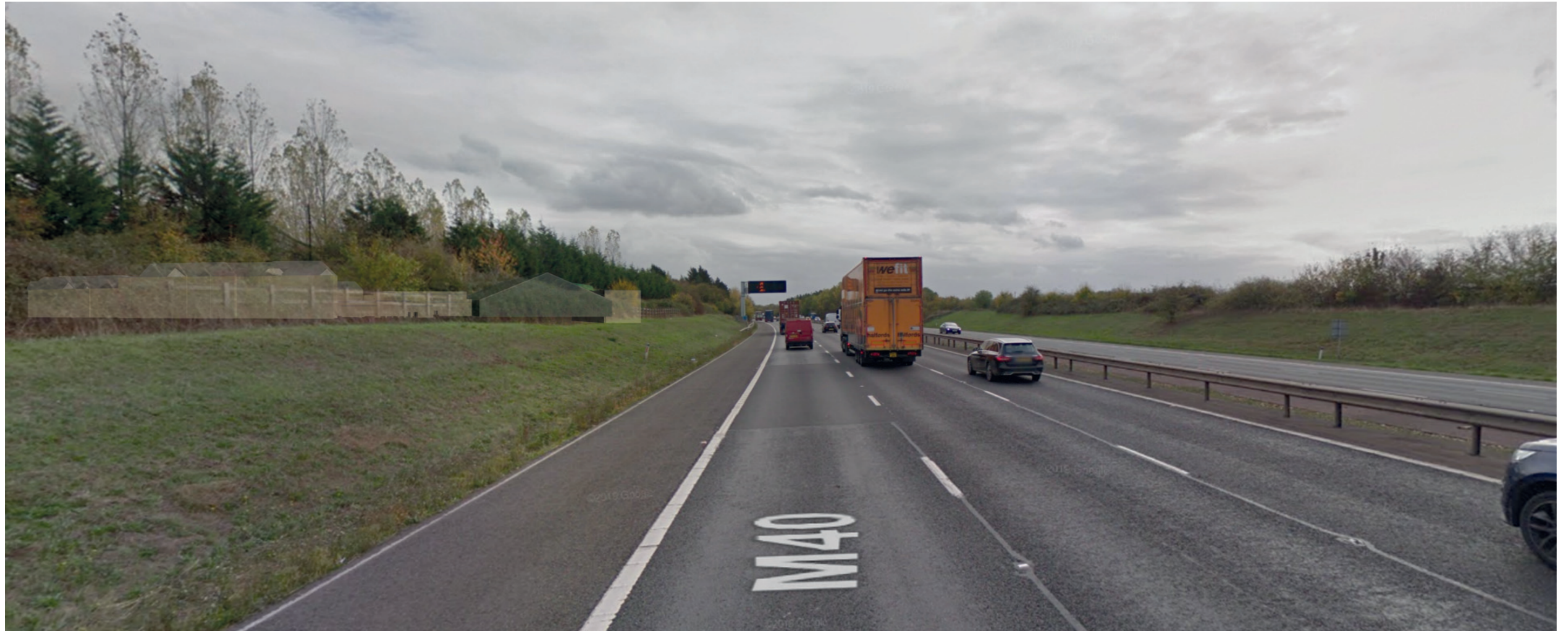
Development not visible in this view, an overlay of the proposed building is shown to indicate its location
