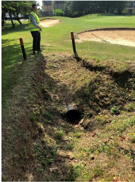
Figure 2-1: Southern Ditch Culvert Inlet
