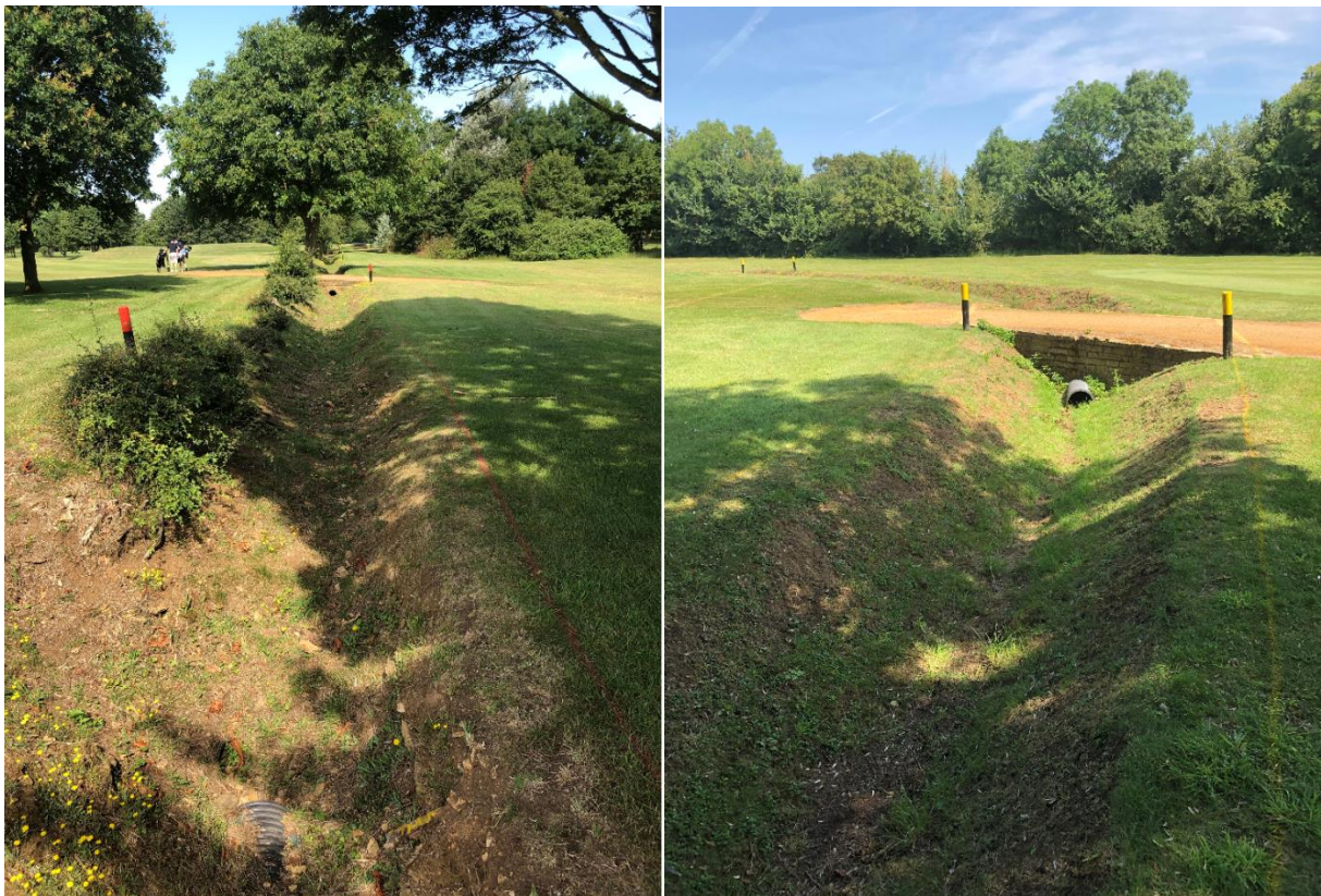
Figure 5-2: Site Drainage Ditches
