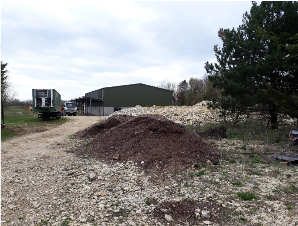
Figure B-3: Excavated stockpiled soils and Limestone recorded off-site.
