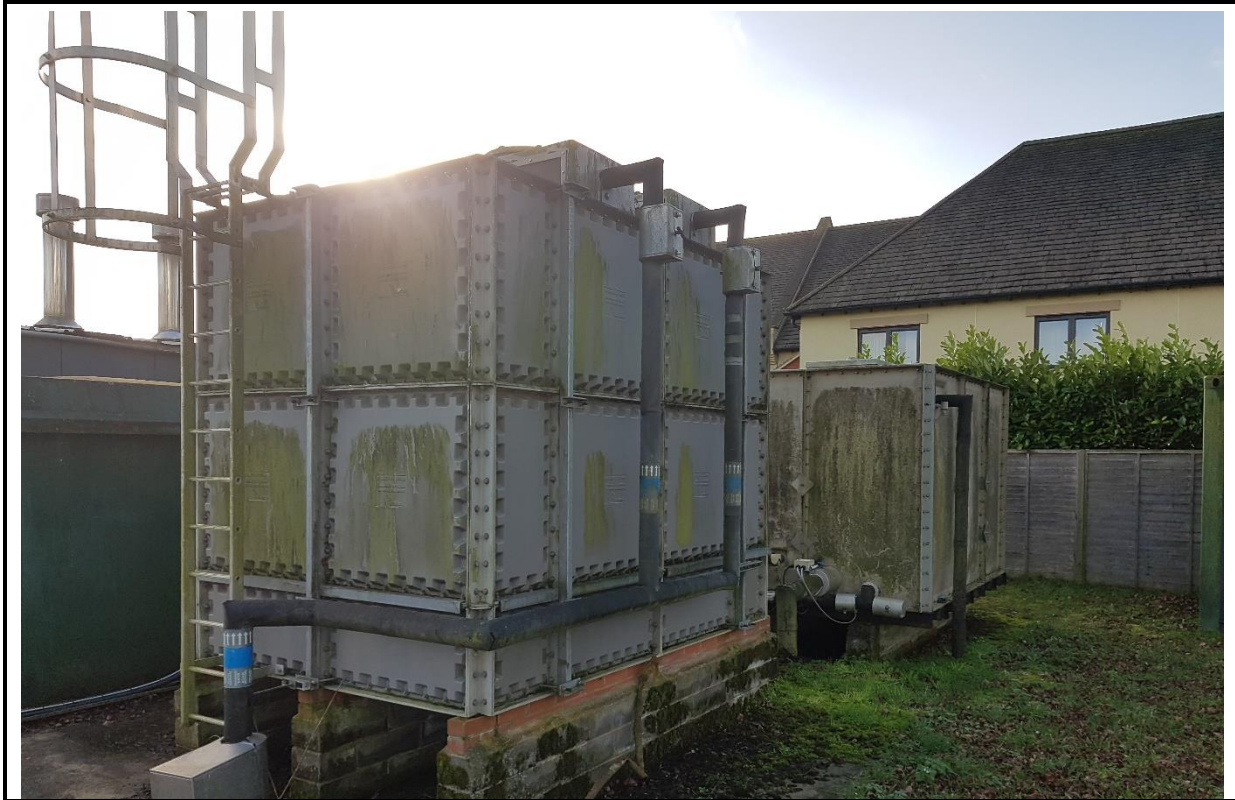
Photo 7: View of the water tanks immediately north of the clubhouse
