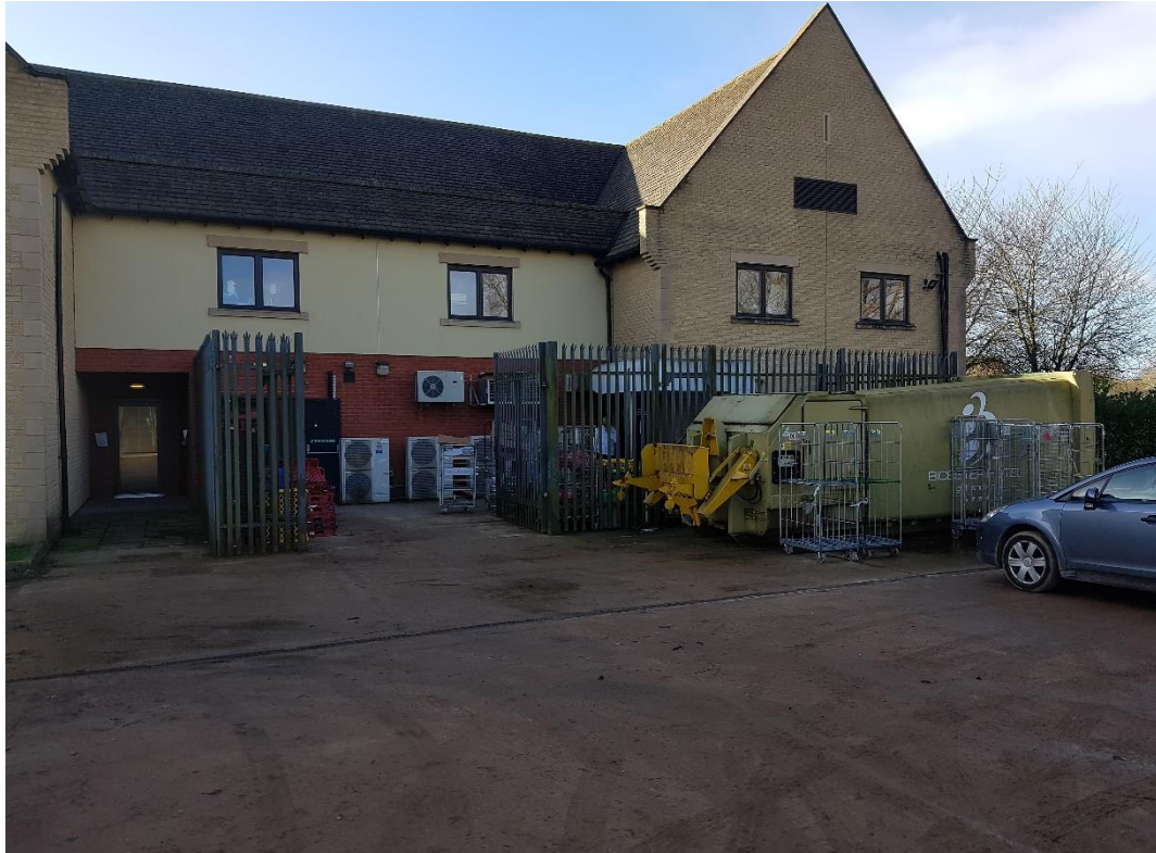
Photo 1: View immediately north of the Clubhouse with air conditioning units and waste compactor
