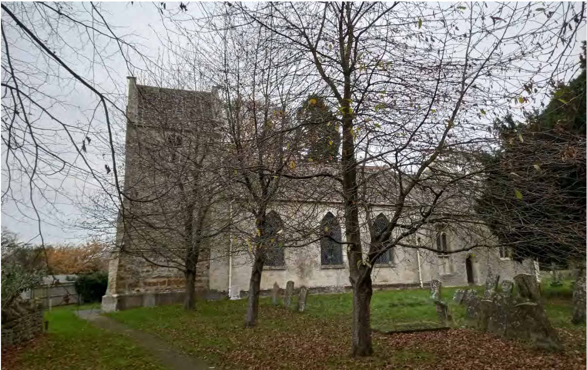
Image EDP A1.16: View north-west towards the Grade II*listed Church of St Mary within the Ardley Conservation Area, illustrating its appearance as well as its surrounding churchyard as an important green space in the conservation area.
