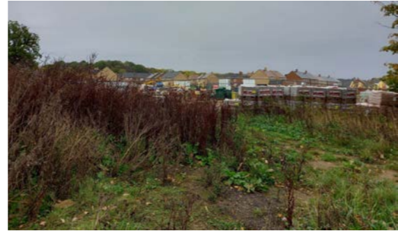
Figure 4: View of the adjacent residential development (Phase 1) under construction
