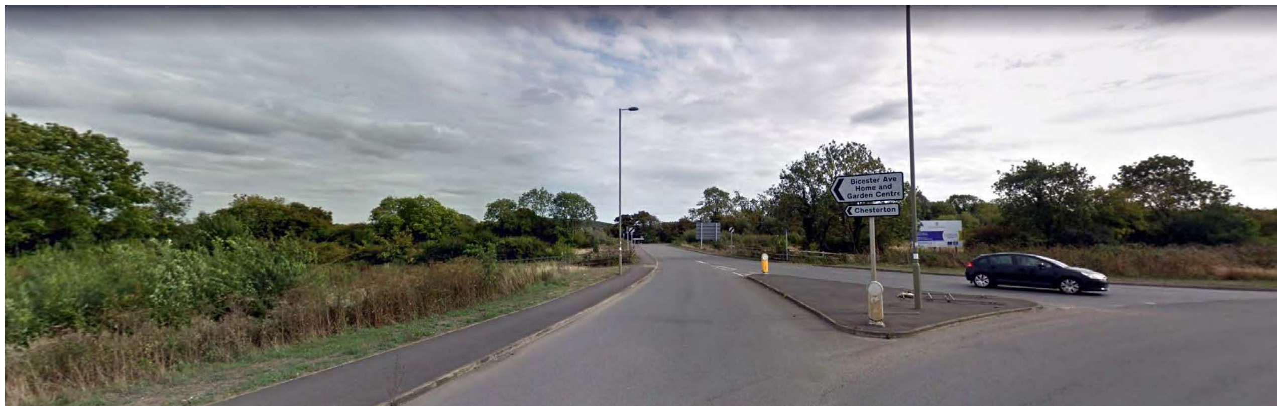
Fig. 12 Looking east along Vendee Drive link road
