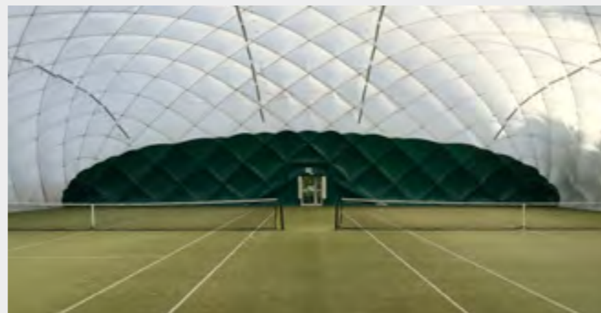
INTERNAL OF TYPICAL AIRDOME
