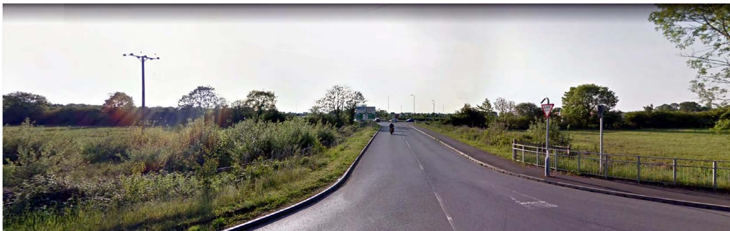
Fig. 13 Looking west along Vendee Drive link road
