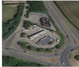
07. Services to A43/B4100 Junction
