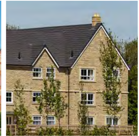
2.5 TO 3 STOREY CORNER BUILDINGS IN STONE AND SLATE TO MARK GATEWAY SPACE
