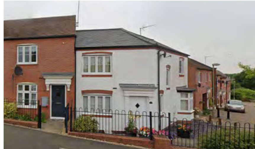
↑ Hanwell Field - Informal frontage with buildings stepping down to follow the contours.*
