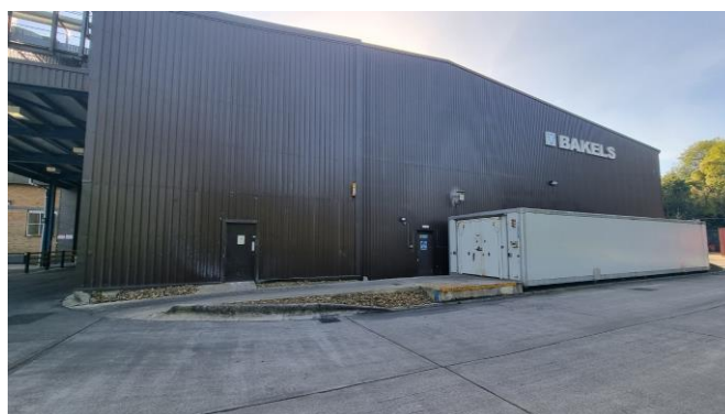
Existing fridge unit to be replaced with boiler enclosure
