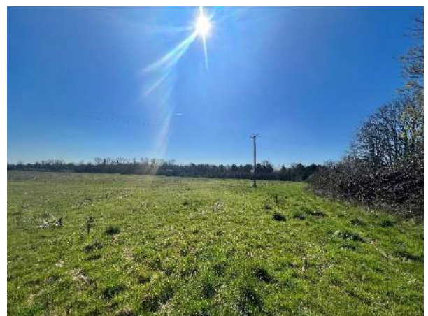
Figure 2.4: Overhead power cables running south-east to south-west and south-west to north-east.
