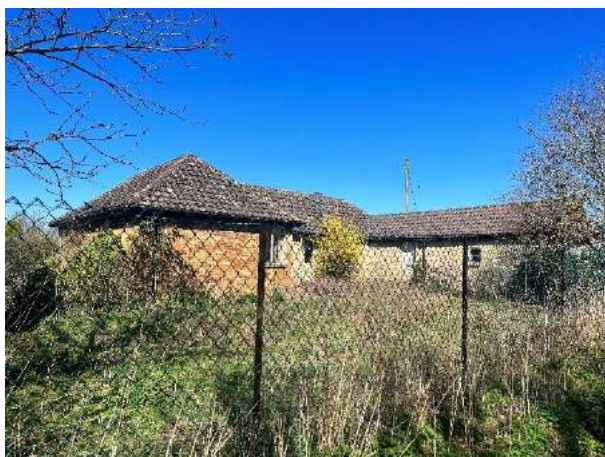
Figure 2.3: Derelict house to the south of the site.
