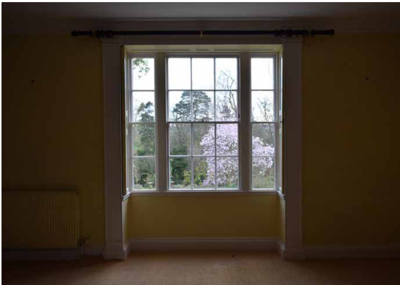
Fig 39: Interior photograph from the living room, looking south into the garden through the 8 by 8 sash windows
