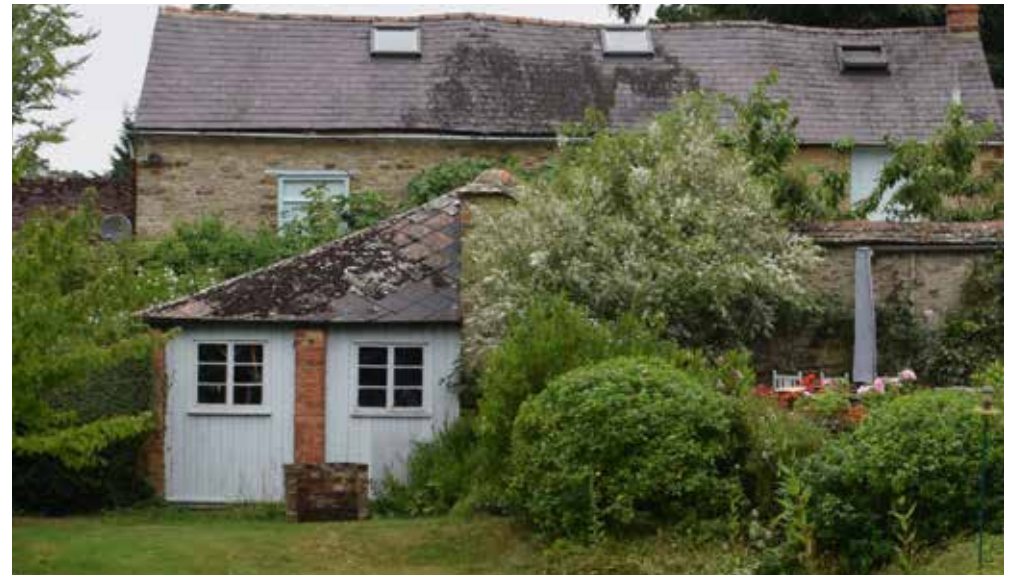
Fig 27: View looking west from the garden showing the rear brick wall and brick piers with timber infilling of two bays.
