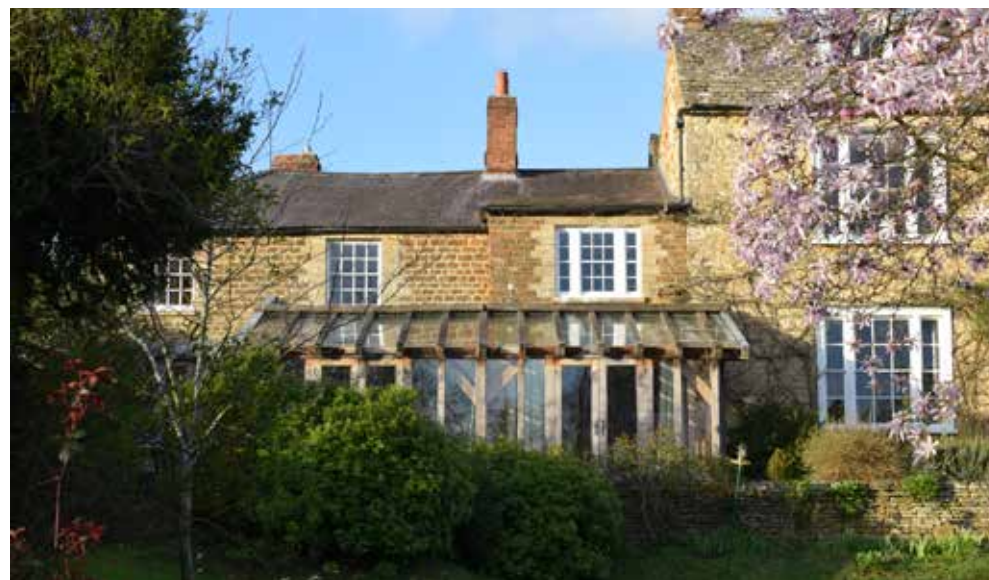
Fig 24: View of the rear (south) elevation of the former service wing showing the 8 over 8 sash windows to the first floor casement to the ground floor on the north wing
