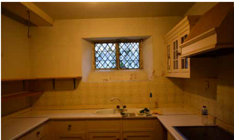
Fig A3.4: Utility room which it is proposed to combine with the boiler room with the removal of the dividing wall. Existing door to be blocked and access via the door into the boiler room
