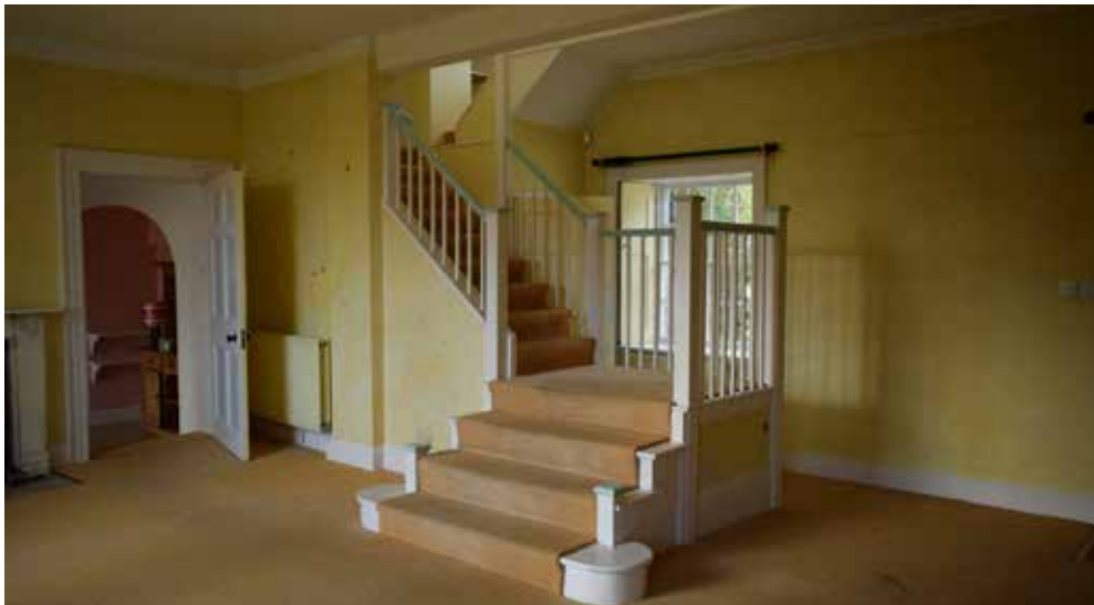
Fig 28: Reception hall showing the wall removed between the back-reception room and service corridor (entrance to which lies behind the staircase dating 1956-86). Also note the new door opening between the reception hall and the kitchen immediately right of the fireplace, also from 1956-86 (the door surround and door reused from the removed hall wall). Line of original wall noted to the left of the pilaster column adjoining the staircase. The removal of the wall and the creation of the opening removed the prior physical and visual separation and distinction between the main house and the former service wing.
