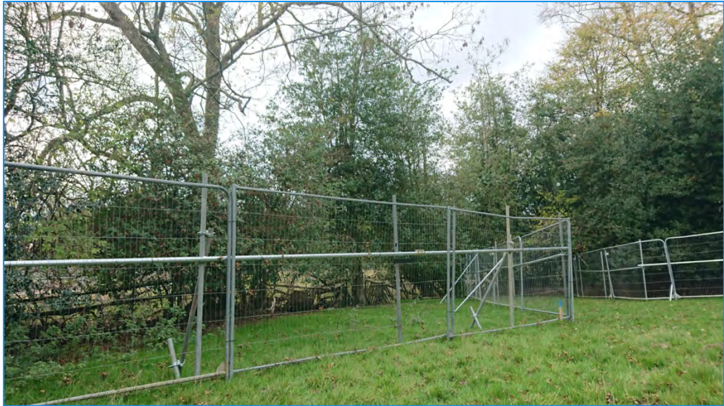
Typical tree protection barrier construction
