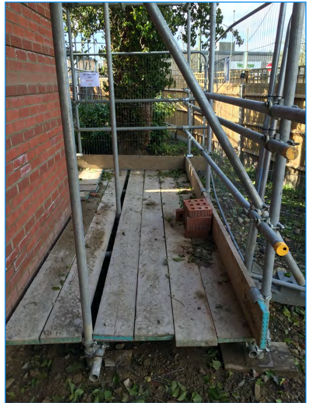
Scaffold ground protection
