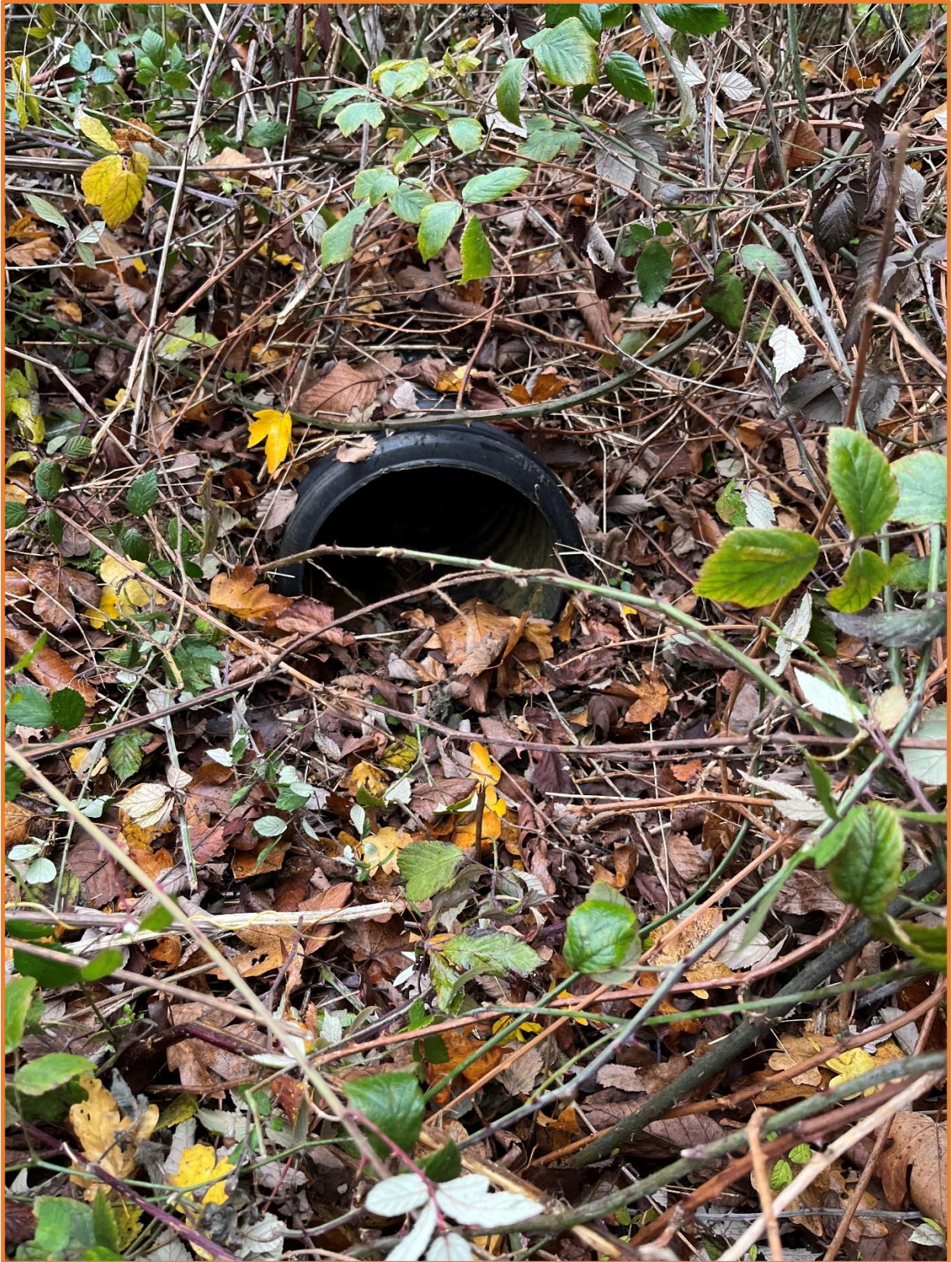
Figure 6: Southern ditch culverted beneath field entrance
