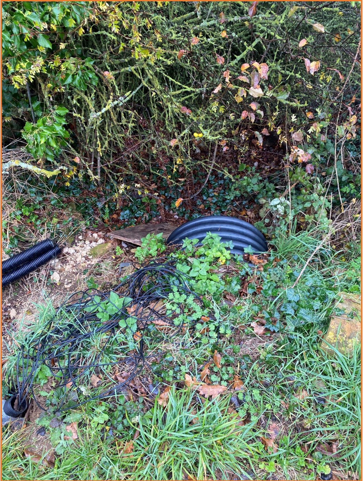
Figure 2: Eastern ditch culverted beneath field access
