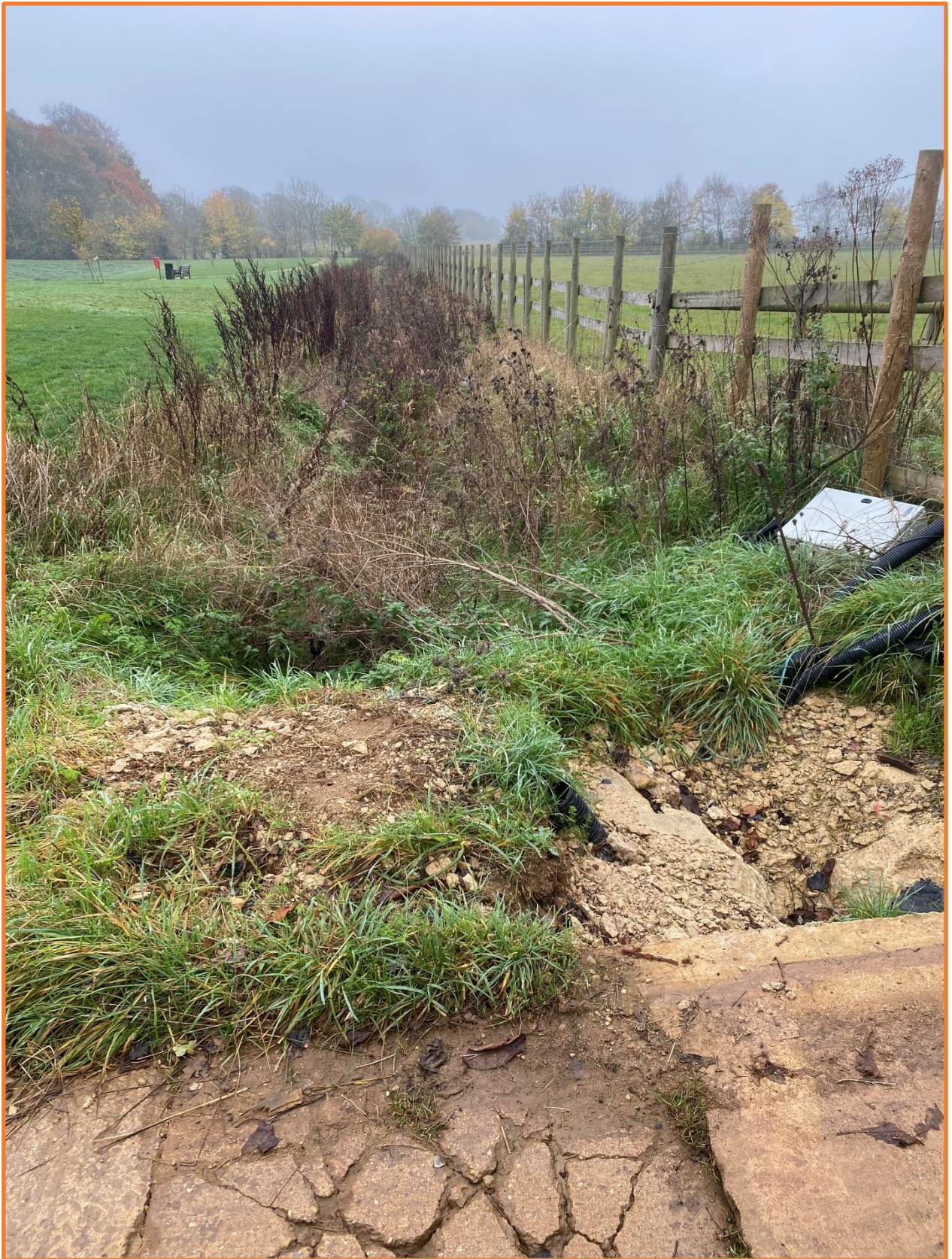
Figure 1: Ditch adjacent to site's eastern boundary
