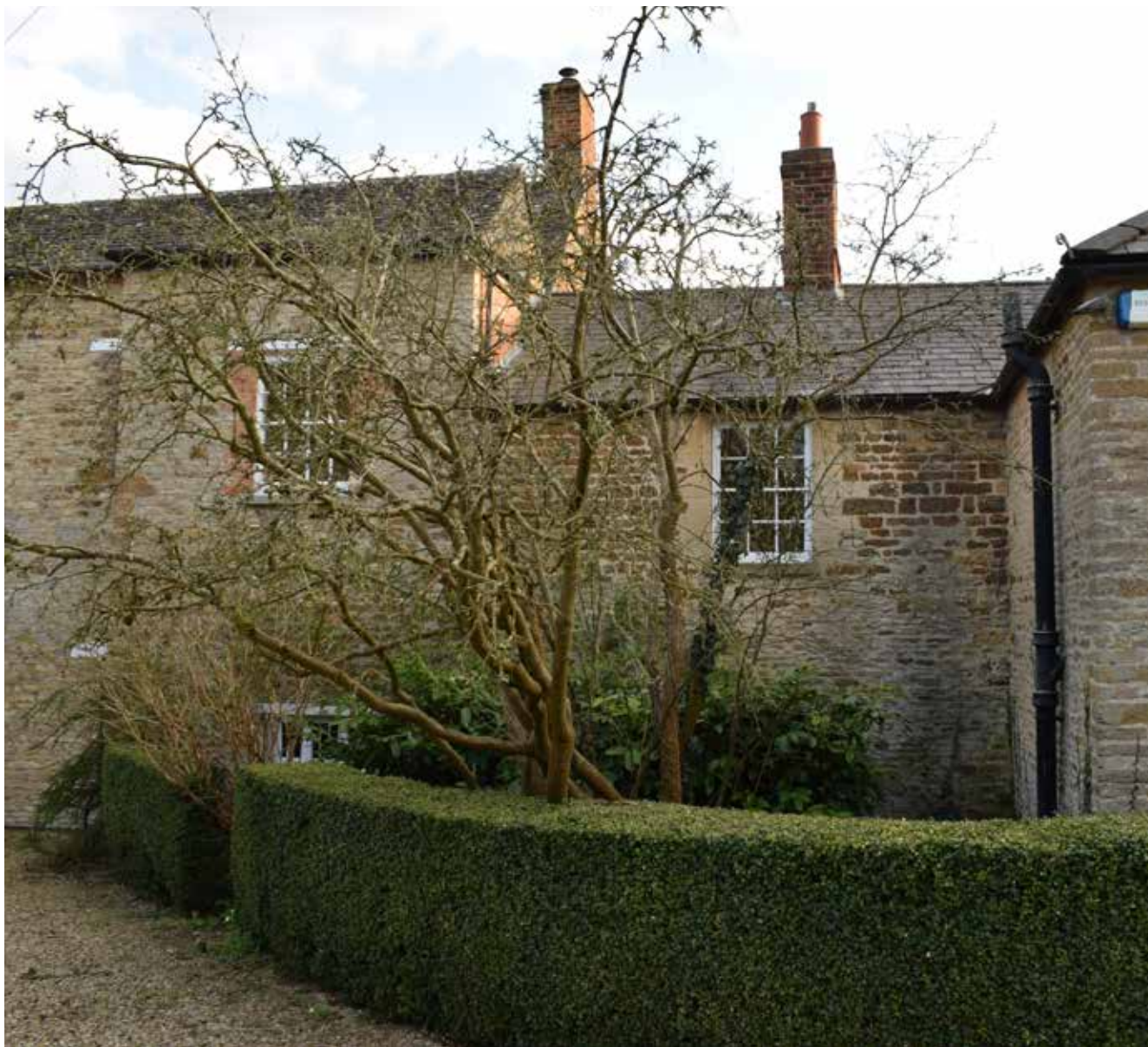
Fig 2: View of the north (front) elevation of Cedar Lodge showing the connection between the main range and the altered and extended service range
