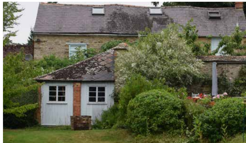
Fig 25: View looking west from the garden showing the rear brick wall and brick piers with timber infilling of two bays.
