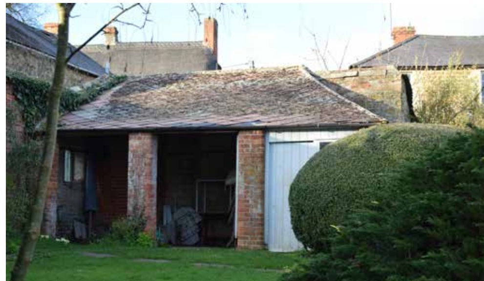
Fig 24: View of the potting shed from the garden looking north showing three sections divided by brick piers with the eastern section enclosed and the hipped roof. The gable roof sits against a brick wall which has a door and a window into the end bay
