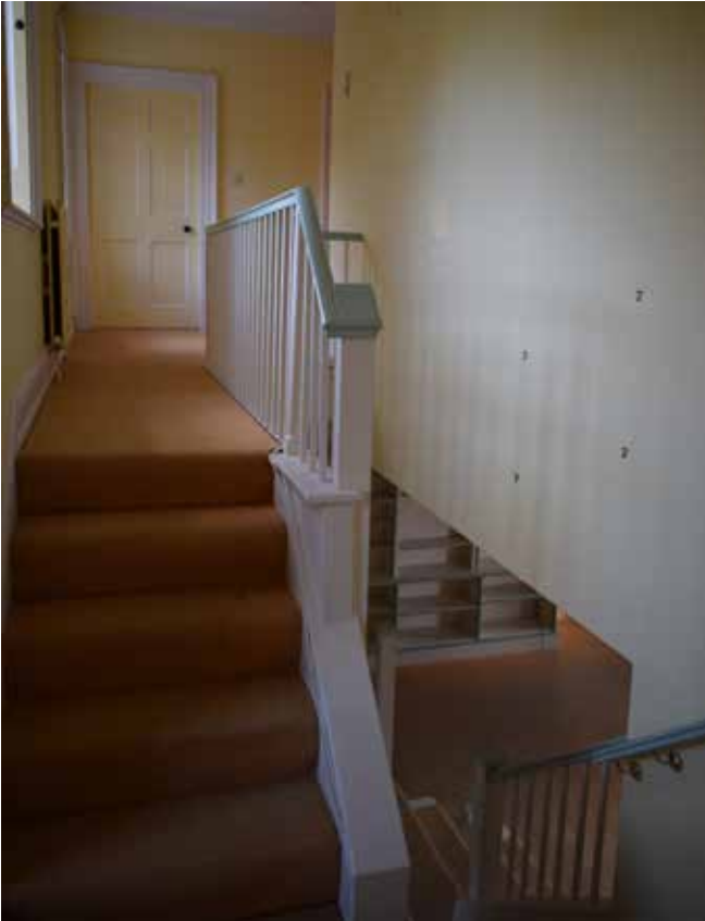
Fig 30: View of staircase first floor balustrade, with late 18th century detailing, which is considered to be original with the 1956-86 alterations. Staircase links through to the former service wing
