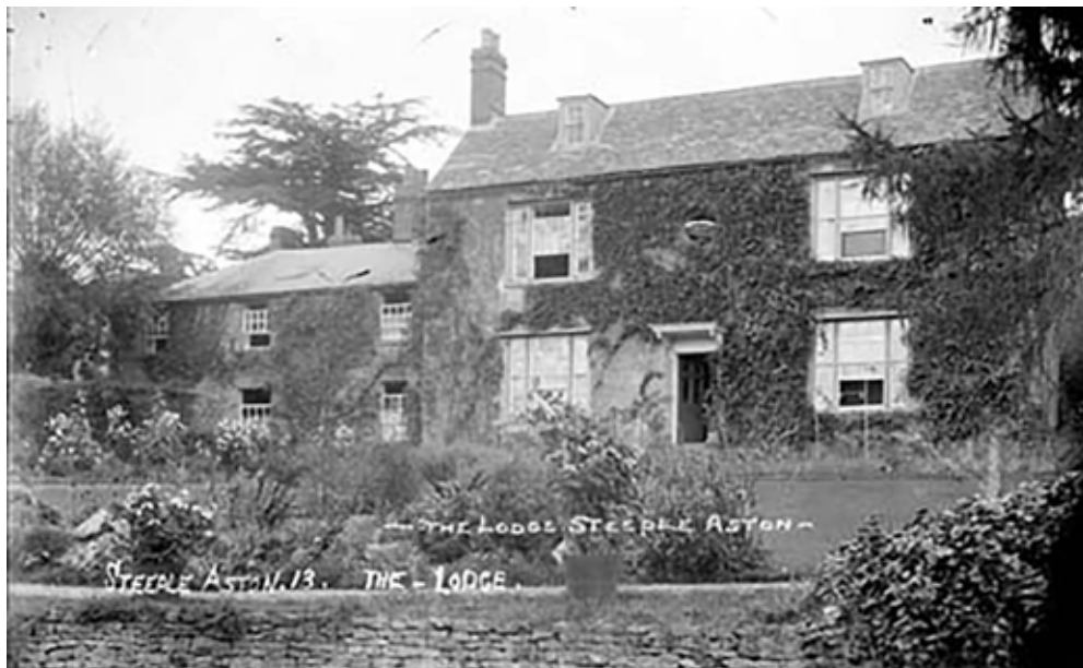
Fig 12: Packer Collection, Oxford History Centre. Photographed c. 1900 – Note tall dormers to the south roof slope and no bay to the ground floor of the service (west) wing with extension above. Elevation appears rendered – list description refers to stucco
