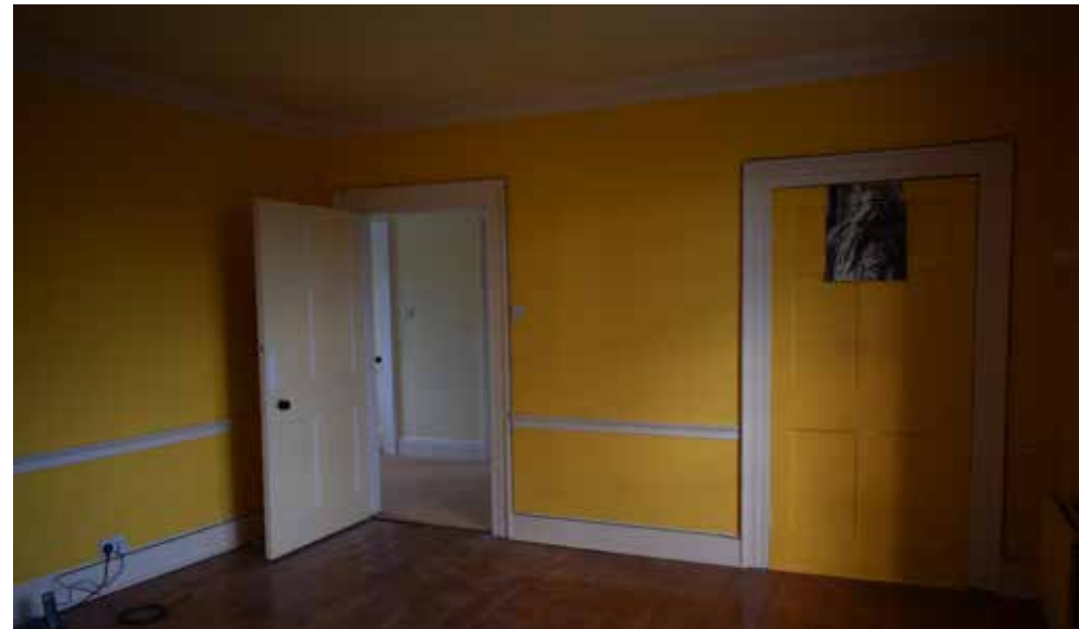
Fig 34: Eastern wall of the bedroom with the entrance door and a door to a narrow cupboard simple skirting, dado and cornice
