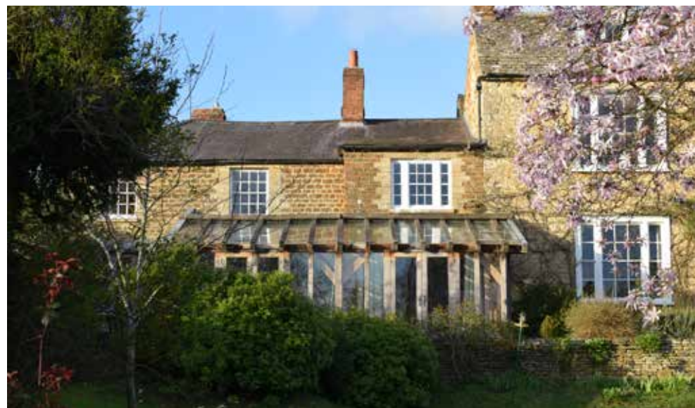
Fig 22: View of the rear (south) elevation of the former service wing showing the 8 over 8 sash windows to the first floor casement to the ground floor on the north wing
