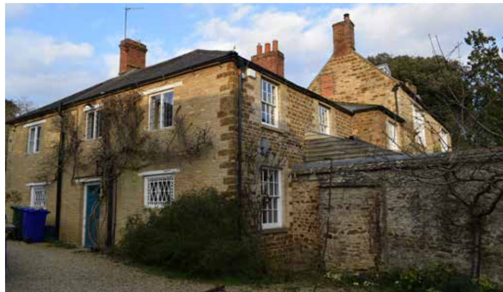
Fig 21: View of the former service wing from the south west showing the symmetrical west elevation of the north south range with the wrought iron casement windows, and the rear (south) elevation with sash windows and the lean-to extension, and the roof of the conservatory over the wall running south west from the elevation.
