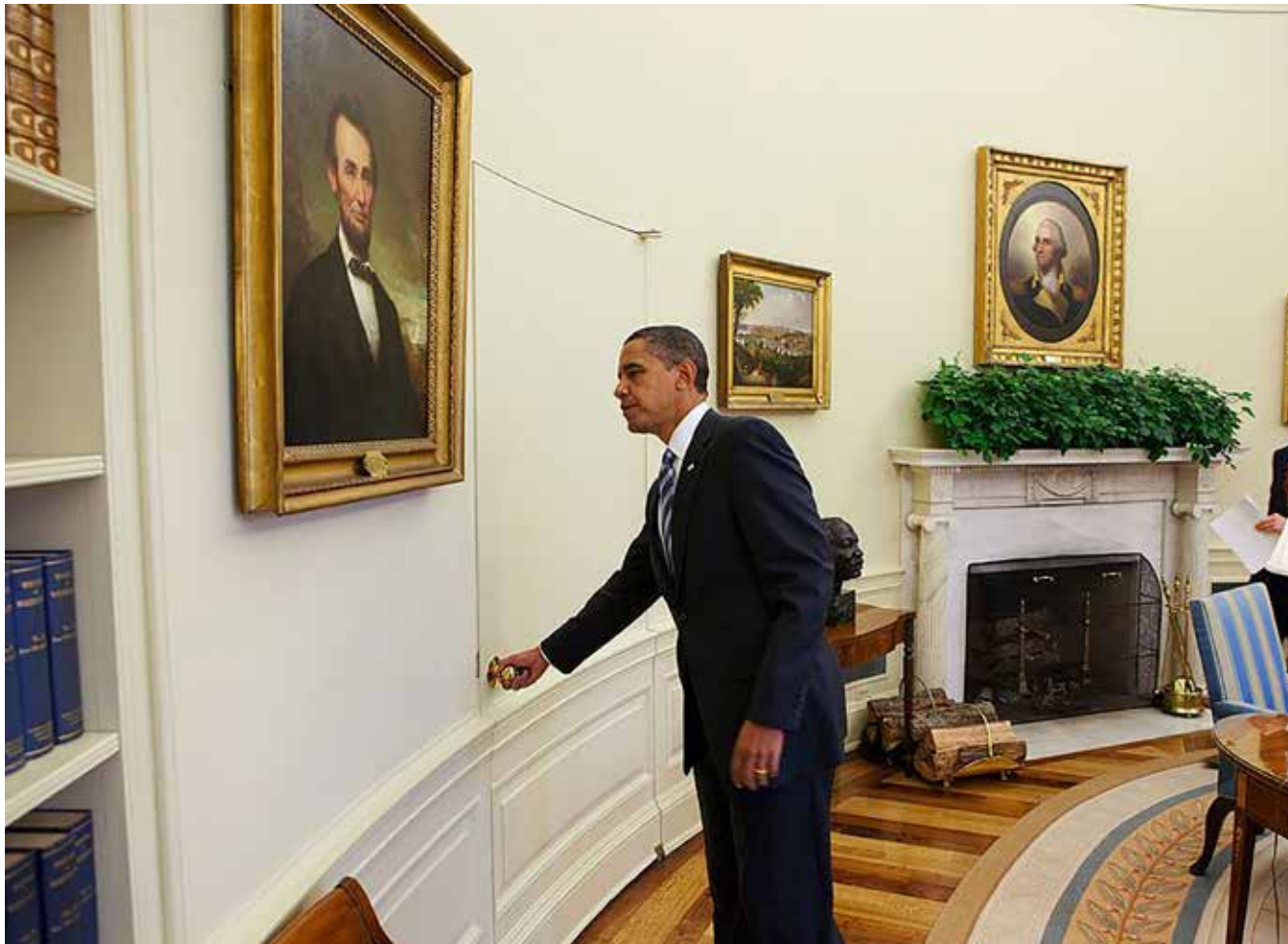
Fig A3.6: One of two concealed or 'jib doors' either side of the fire place in the Oval Office, at the White House
