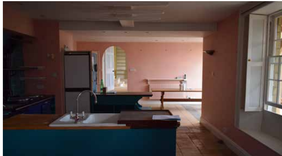
Fig 28: Kitchen dining room in the former service wing showing the opening created during the 1956-86 period which joined the main reception room directly into the former service wing thus avoiding the need to enter via the historic link running along the south side of the house. Also shows the opening created by the removal of a later bay wing to gain access to the conservatory added 2001. This area is much altered
