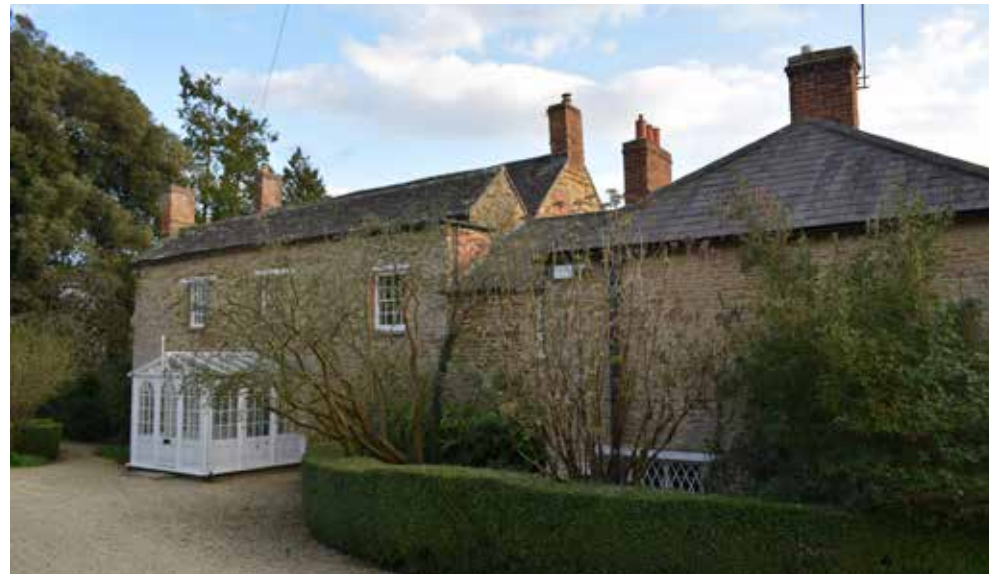
Fig 18: North elevation from the northwest showing the main range with modern timber porch the two-storey extension and the former service wing
