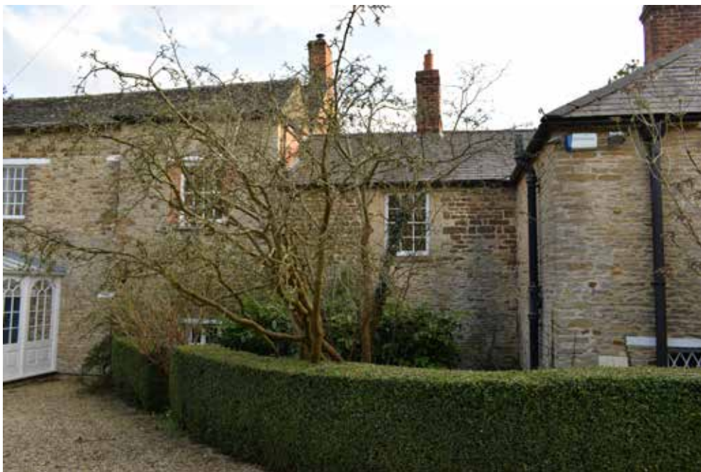
Fig 22: View of the former service wing with the link to the north-south range with timber sash to the first floor of the link and a metal casement to the ground floor on the north wing
