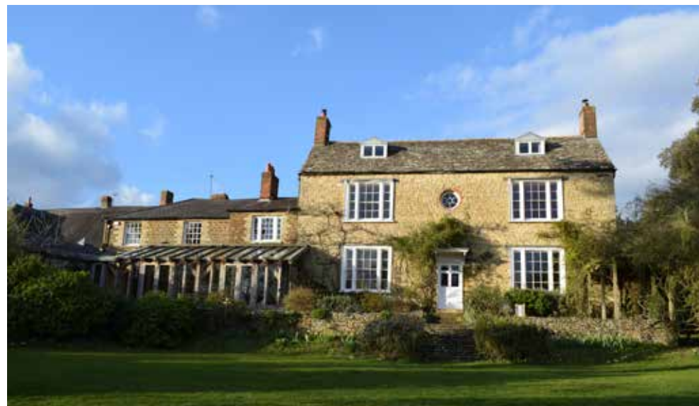
Fig 21: Rear (south) elevation of the house with symmetrical elevation and former service wing to the west with new conservatory and reintroduced dormers to the roof.
