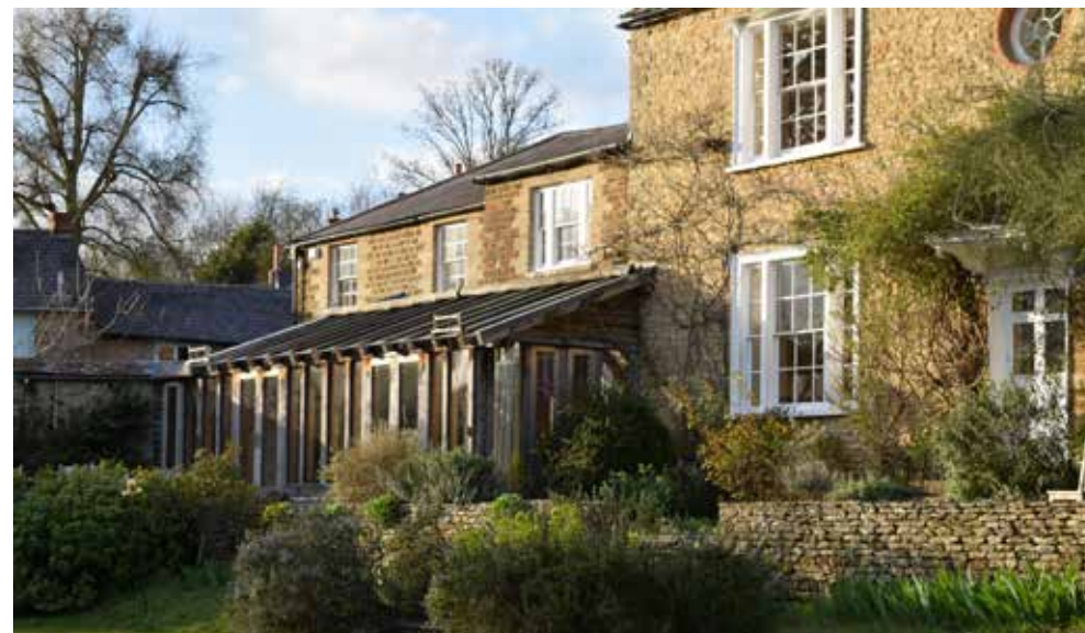
Fig A3.10: 2001 conservatory which is to be demolished and replaced by a new kitchen extension
