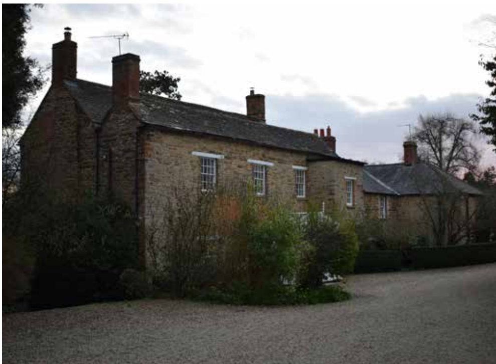
Fig 19: North (front) elevation of the house from the northeast showing asymmetrical gables, front elevation of the main range with the two-storey projecting c. 1860s extension and former service wing to the west
