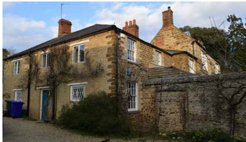
Fig 23: View of the former service wing from the south west showing the symmetrical west elevation of the north south range with the wrought iron casement windows, and the rear (south) elevation with sash windows and the lean-to extension, and the roof of the conservatory over the wall running south west from the elevation.
