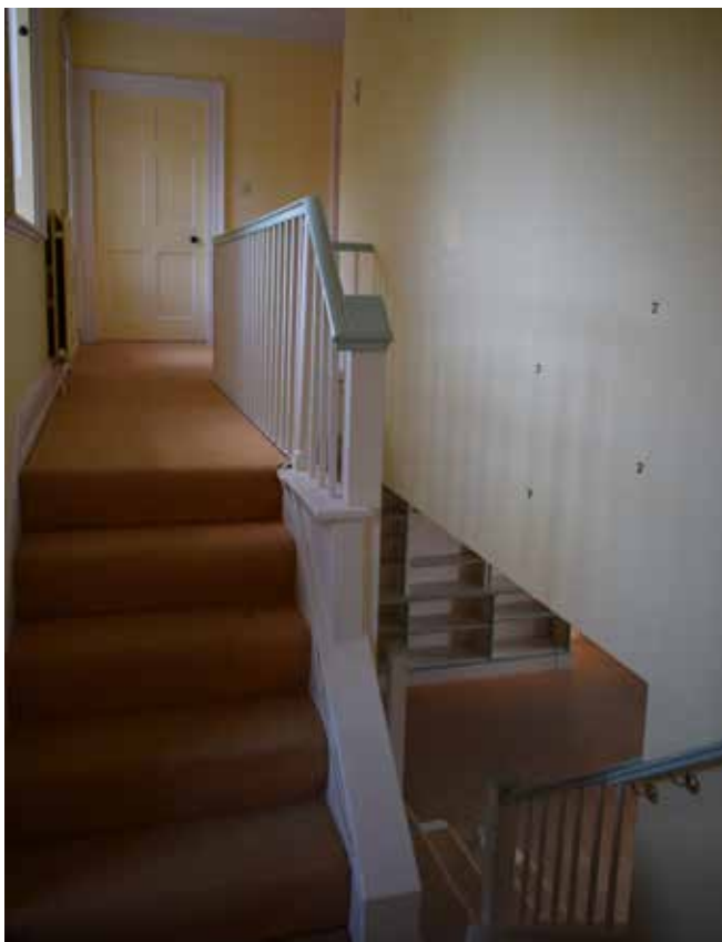
Fig 32: View of staircase first floor balustrade, with late 18th century detailing, which is considered to be original with the 1956-86 alterations. Staircase links through to the former service wing
