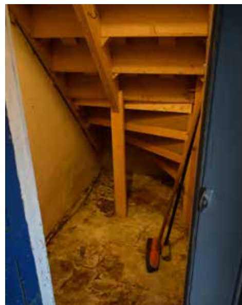
Fig A3.6: The stair in the service wing which appears to have been recently replaced. Proposal is to remove and install a new, compliant stair in this location
