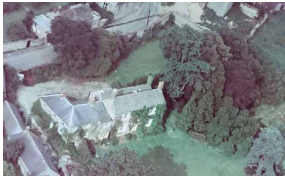
Fig 14: Aerial image c1970 (Sava Report 2013) showing house and grounds when occupied by Iris Murdoch and John Bayley. Note no dormers to the south roof slope
