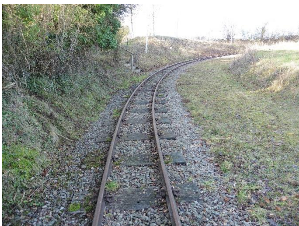
Photo 5: Railway line with edges of ephemeral vegetation.
