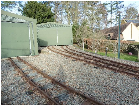
Photo 9: Area of track ballast south of the storage buildings.
