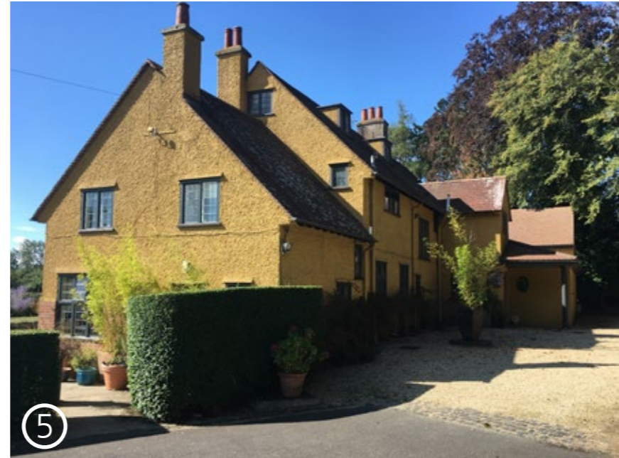
Existing Dwelling House
