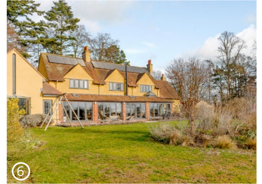
Existing Dwelling House
