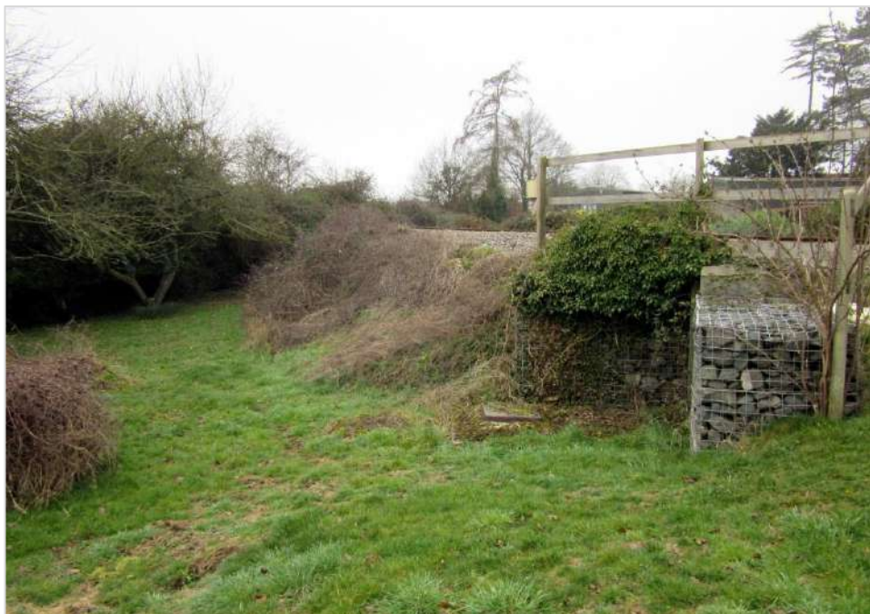
Image 4: The railway track running on an embankment around the southeast side of the garden.
