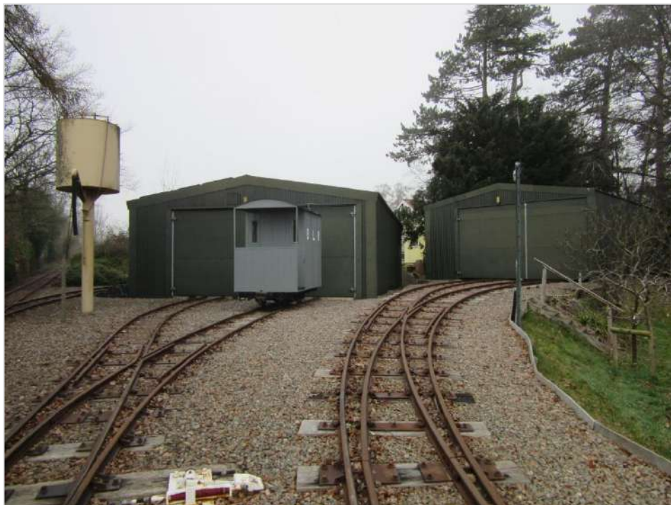
Image 6: Engine sheds situated on the southwest and west sides of the house.
