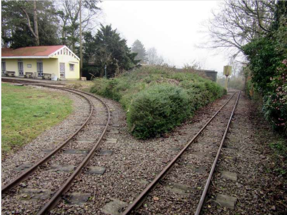
Image 7: Looking east-southeast, showing the station (left) and the track down to the engine sheds and the southeast angle of the site (right).
