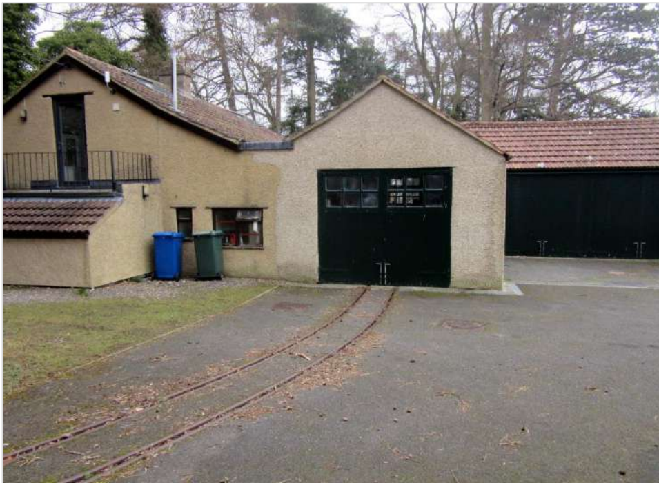
Image 2: Outbuildings northeast of the house.
