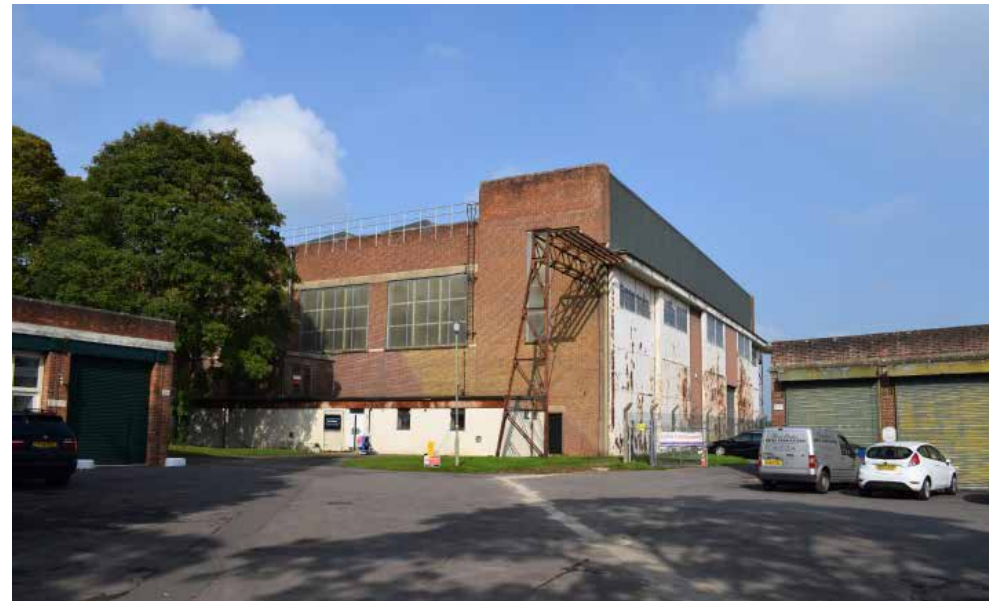
Fig 18: Northern most C Type Hangar
