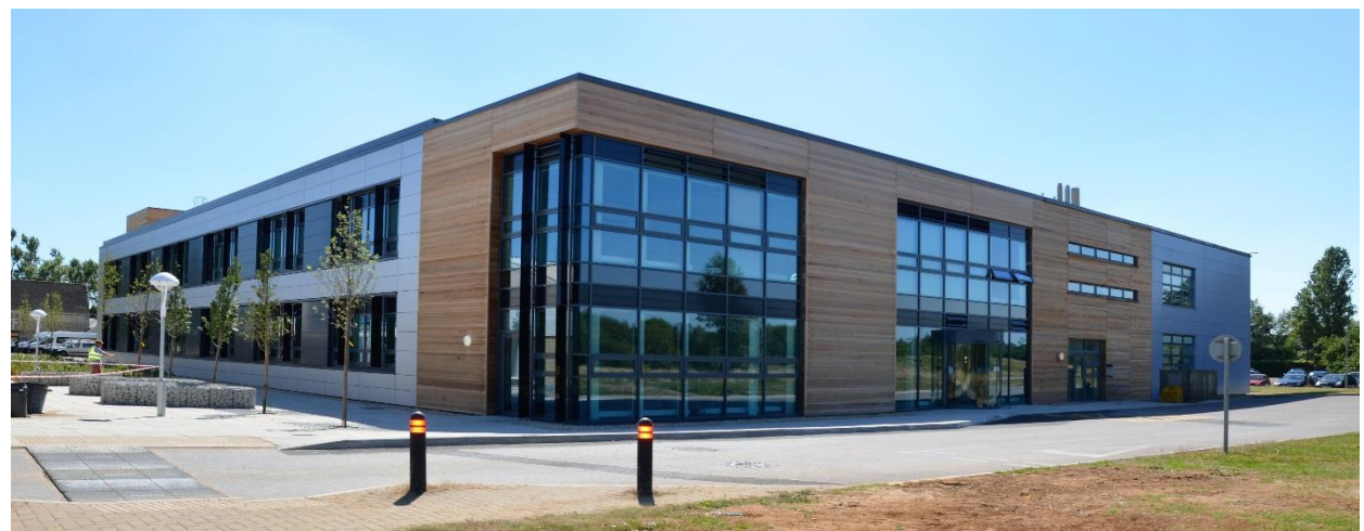
Figure 2: Centre for Innovation & Enterprise Extension
