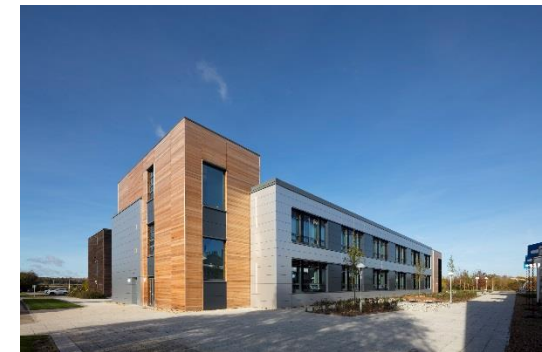
Figure 11: Timber cladding highlights vertical features
