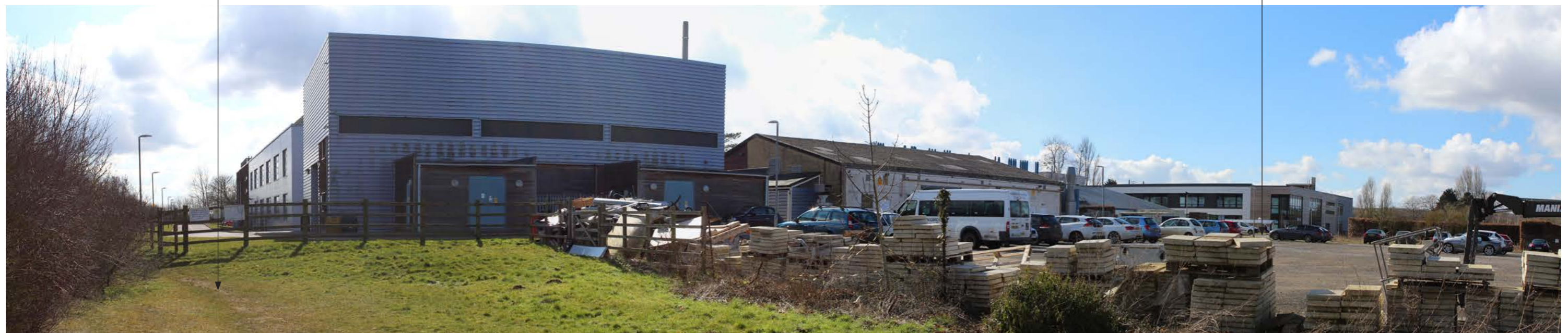
PHOTO VIEWPOINT I: View southwest from public footpath north of the IAT building (Institute of Advanced Technology)
