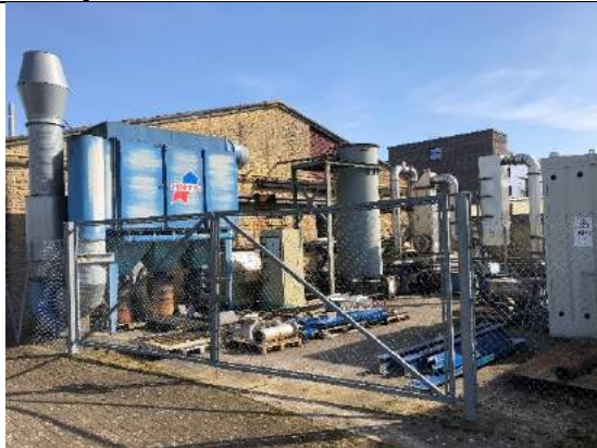
Plate 11: Rear of main facility
