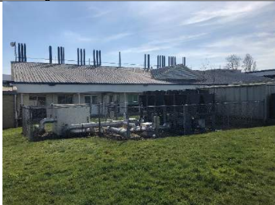
Plate 12: Rear of central building
