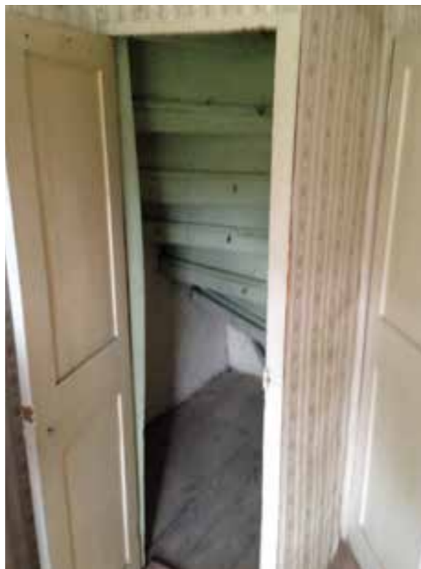
Existing steep winder staircase carcass is in a fair condition
