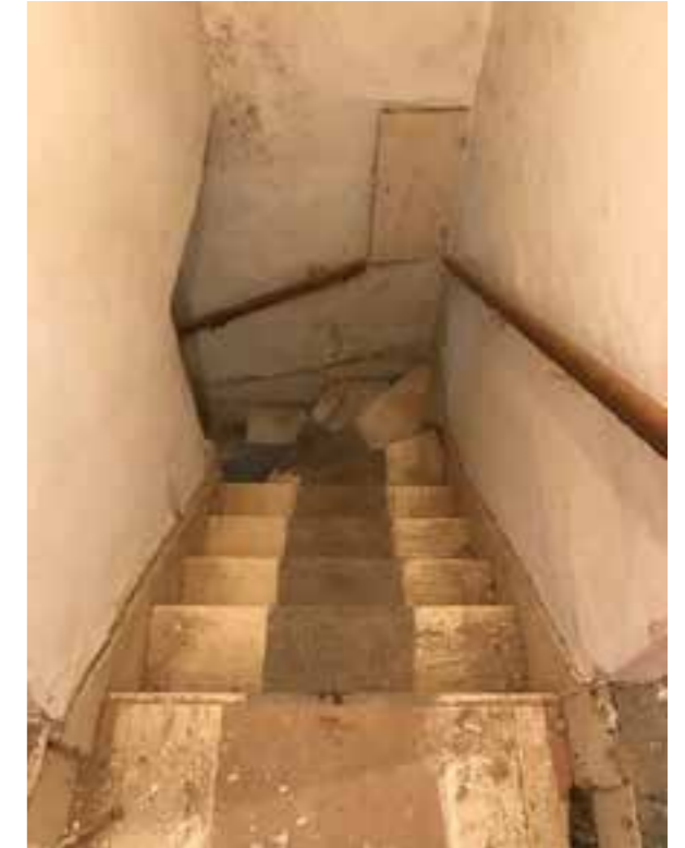
Existing Timber Stairs
