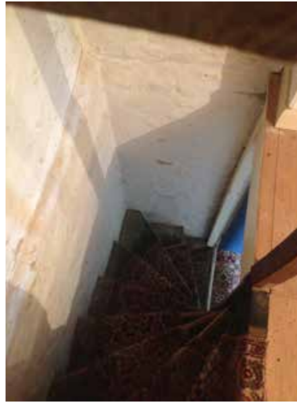
Existing steep winder staircase
