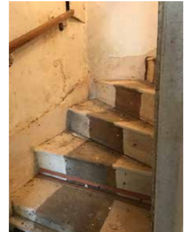
Existing Timber Stairs
