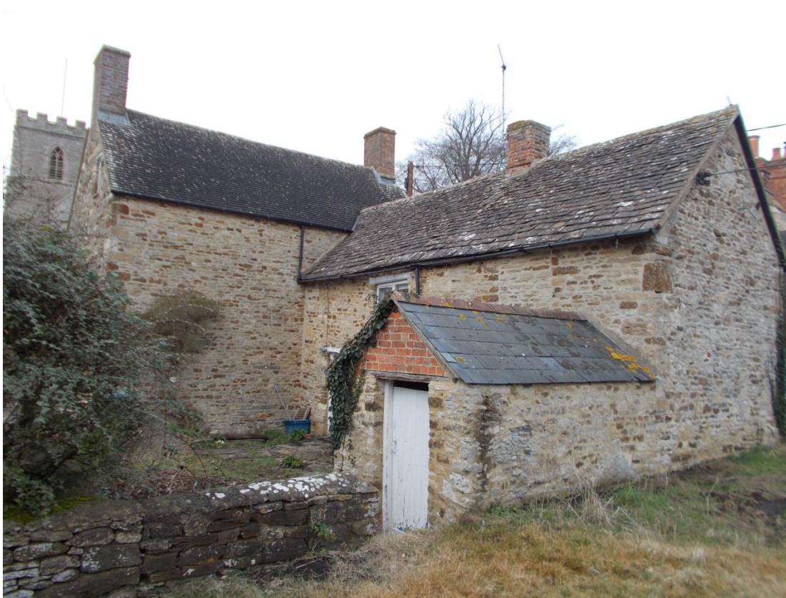
Photo 3 – rear elevation from east
