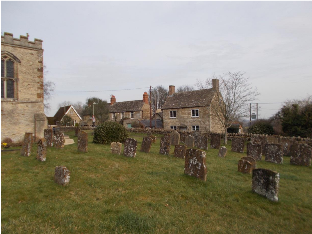
Photo 9 – from west church yard
