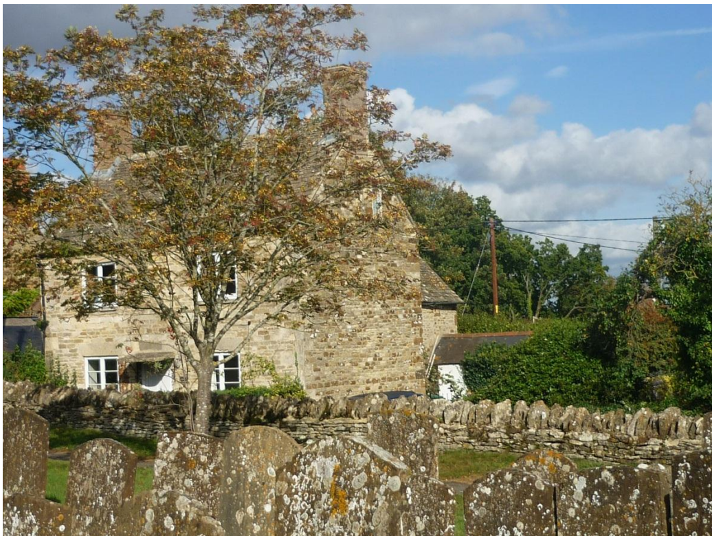
Photo 10 – from west church Yard
