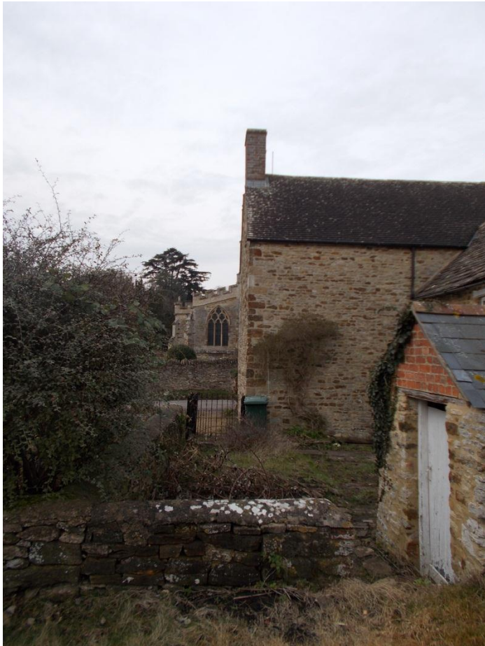
Photo 5 – from east to rear view of church
