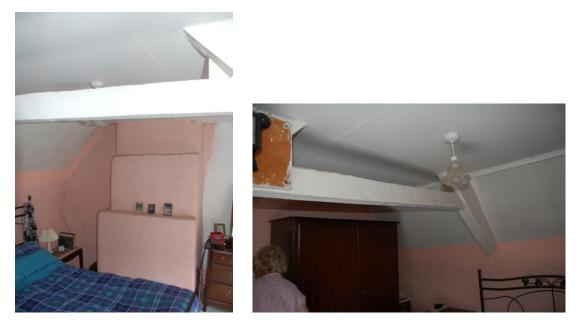
Despite its rather limited headroom, the loft area over the kitchen has long since been converted into a bedroom, accessed from the top of the main staircase. Apart from the exposed rafters, the most striking feature is the stepped chimney-stack at its far end, the brickwork plastered over. This would have radiated considerable heat when the range was alight. It seems unlikely it ever included a fireplace, and this was confirmed (as far as possible) by tapping.
