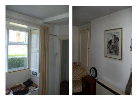
Unlike the main room it has a wooden floor. This room has no visible fireplace, but a deep cupboard in the wall at the SE corner provides some evidence for a blocked chimney-breast in the east wall. This is deeper than the equivalent open recess in the SW corner.
