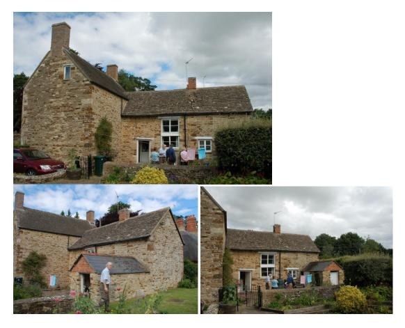
The ground floor of this further extension has now been converted into a bathroom, with a window replacing the earlier doorway. (The left-hand end of its rough wooden lintel set oddly between two of the ashlar blocks). The loft window-opening has been blocked in, but its outline is still visible just left of the roof to the outside privy.
