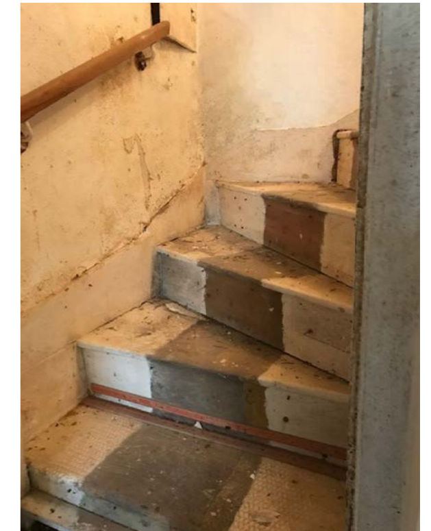
Existing Timber Stairs
