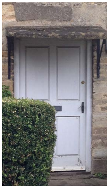
Existing Front Door (Ground floor, front facade)
