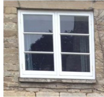
Existing Bedroom Room Window (First floor, front facade)
