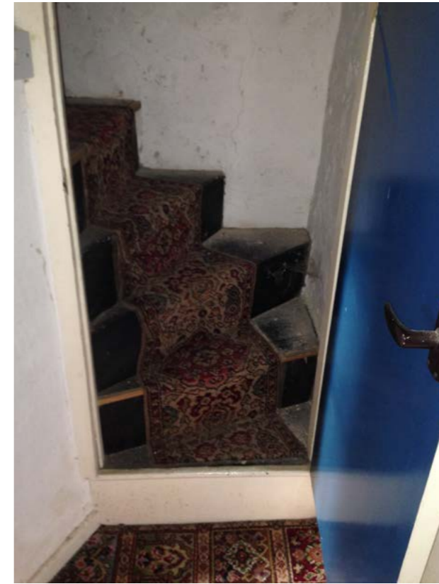
Existing steep winder staircase showing non-original stair treads and door
