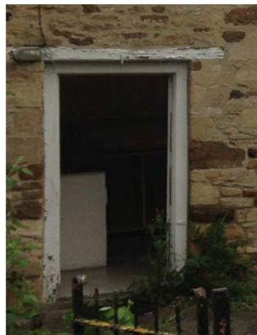
Existing Back Door (Ground Floor. South facade)
