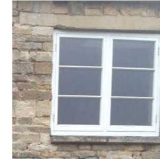
Existing Bedroom Room Window (First floor, front facade)
