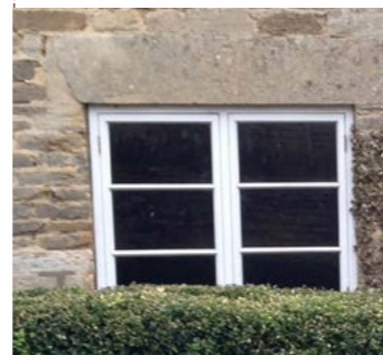
Existing Sitting Room Window (Ground floor, front facade)
