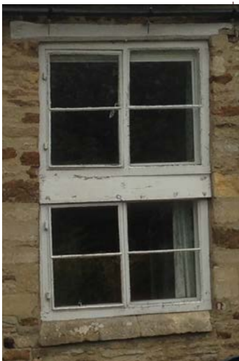
Existing Kitchen Window (Ground floor/ First floor, South facade)
