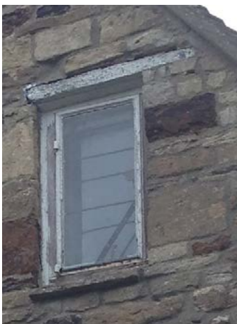
Existing Loft Window (Second Floor. South facade)
