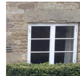
Existing Living Room Window (Ground floor, front facade)
