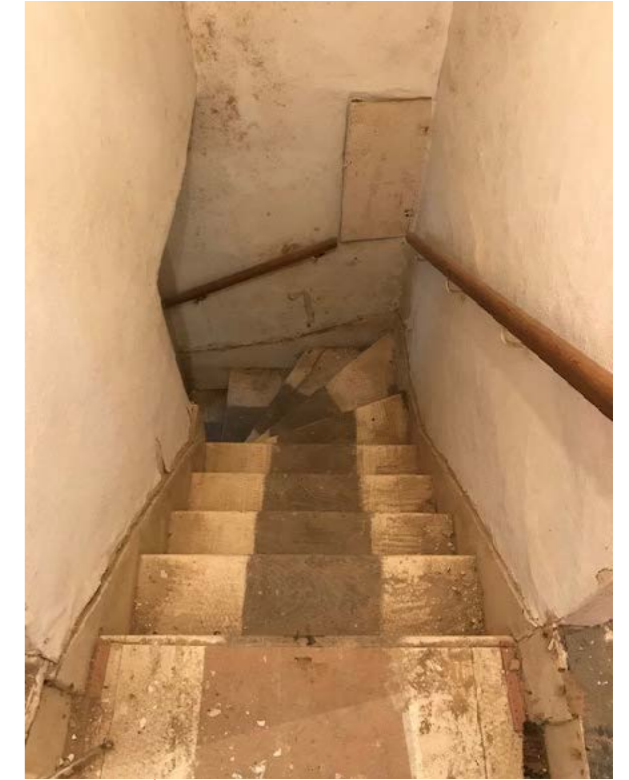
Existing Timber Stairs
