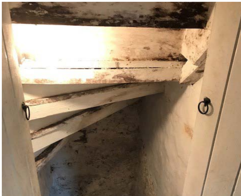
Existing Timber Stairs from below, the black mould from damp ingress into the existing stairs will need to be addressed or removed if the timber is completely rotten.
