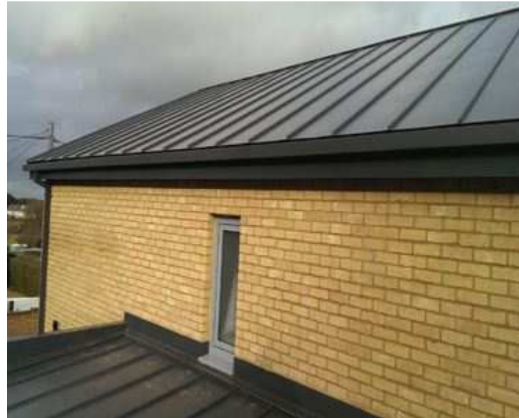
Kalzip Dark Grey Standing Seam Roof
