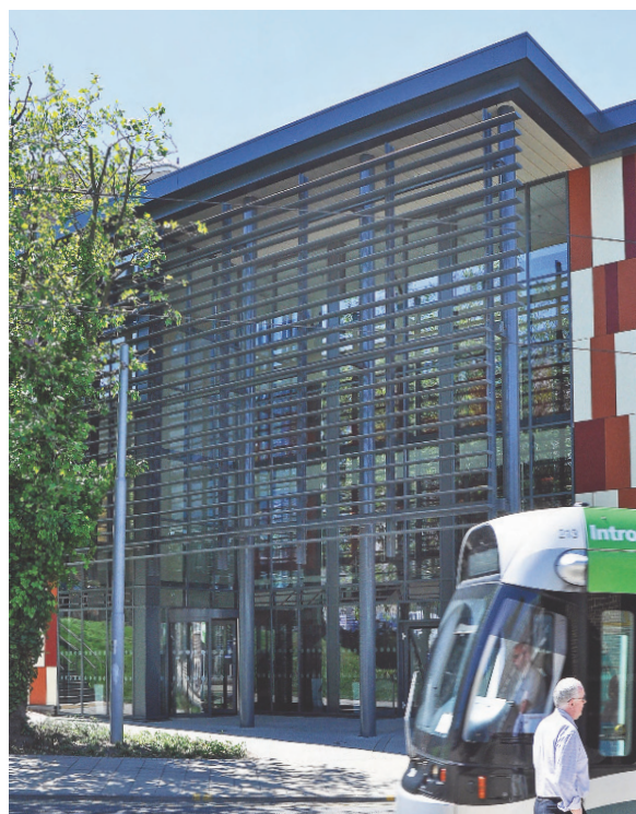
View of installation at Nottingham Trent University.
