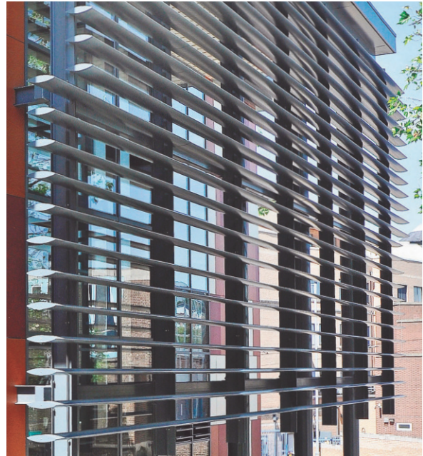
Efficient solar shading without loss of natural daylight and outside views.
